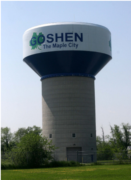
Photo from City of Goshen
