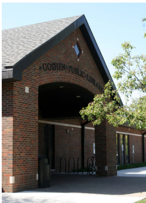
Photo from City of Goshen
