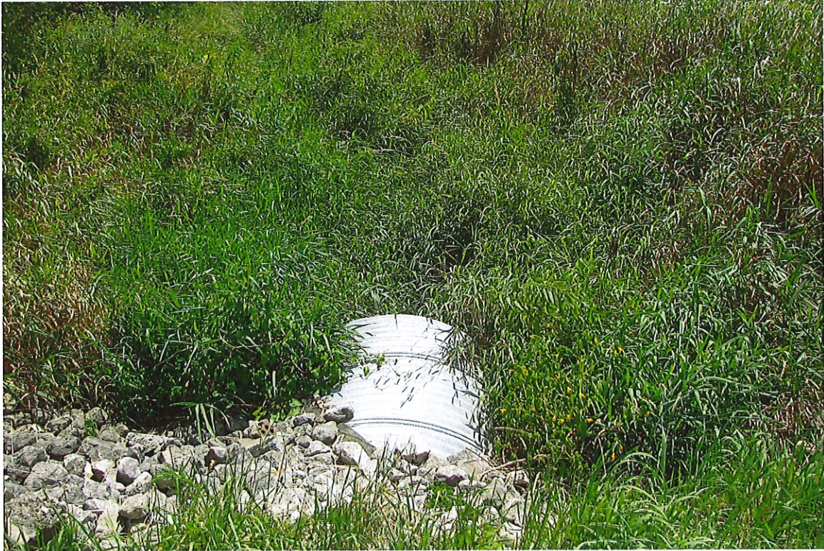
LOW WATER LEVEL AT WEAVER DITCH CR 44 (LOOKING DOWNSTREAM)
