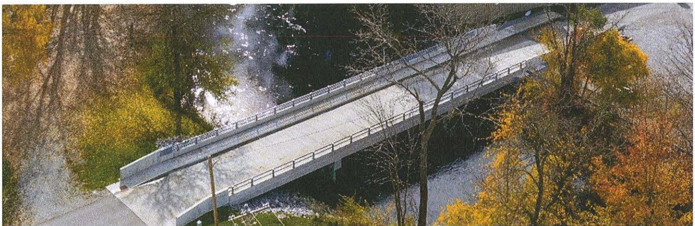
Noble County Bridge 147 over Elkhart River — Three-Span Reinforced Concrete Slab
