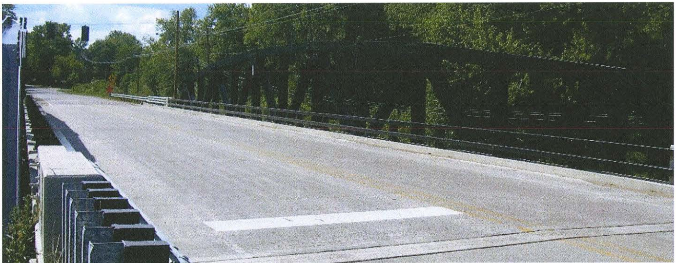
Columbia Road over Grand River, Ingham County, Michigan
