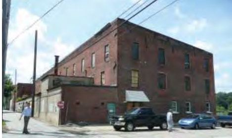
EXISTING MAIN ENTRANCE
