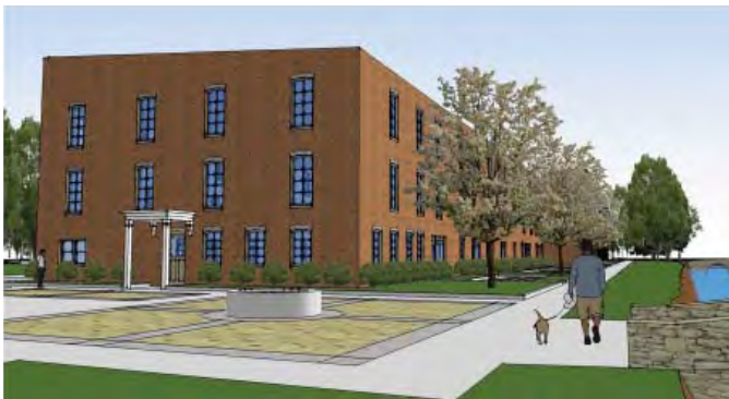
VIEW OF NORTHWEST CORNER ALONG MILL RACE
