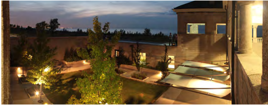
COMPLETED COURTYARD VIEW
