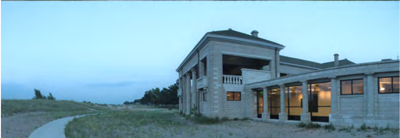
EXTERIOR VIEWS - LAKE SIDE
