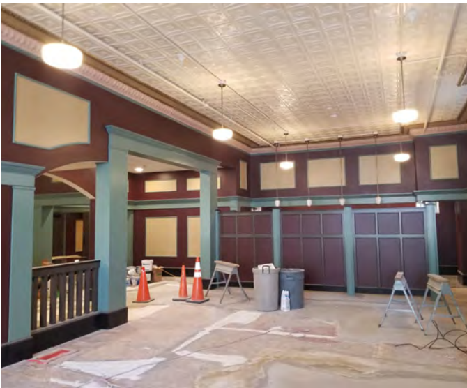
FINISHING TOUCHES ON NEW LOBBY
