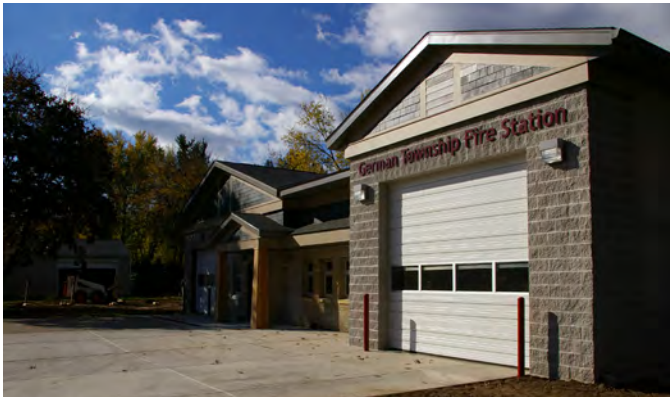
VIEW OF NEW FIRE ENGINE BAY
