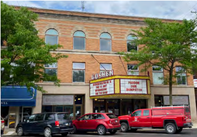
RENOVATED FACADE WITH RESTORED STOREFRONTS
