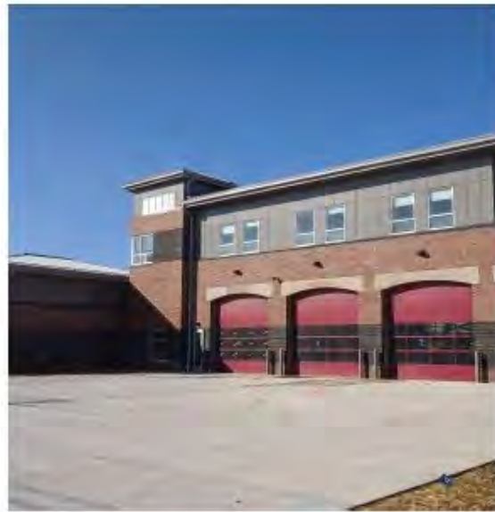
WHITE RIVER TOWNSHIP FIRE STATION Johnson County, IN
