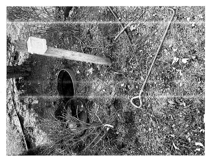
I went out to the Court Yard Condominiums today to see if they qualified for sewer relief. The repair is the gray pvc in the first pic. There is no drain in the bottom of the structure or anywhere close to the manhole lid. They would qualify for sewer relief.
