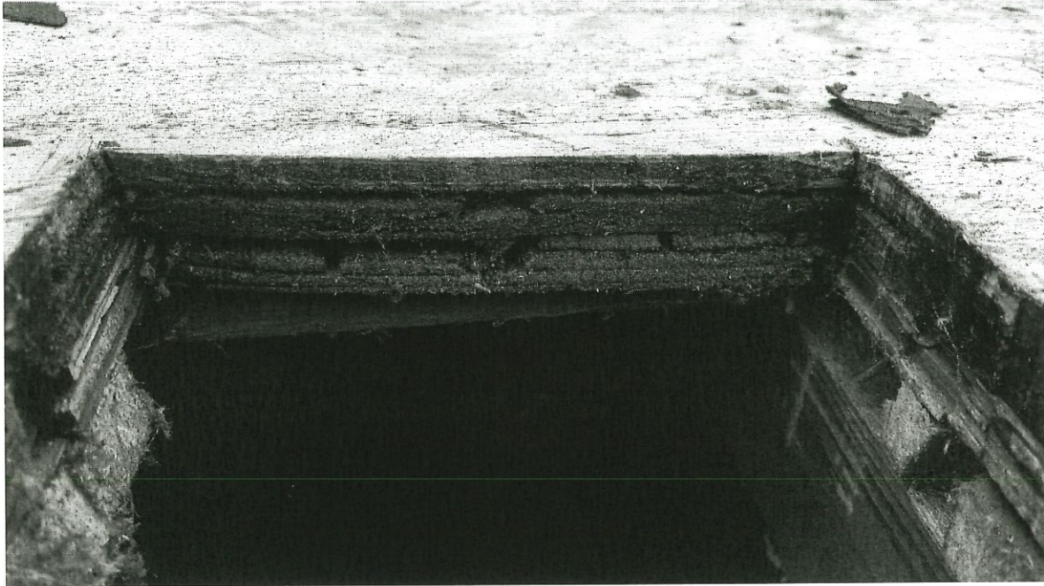
Photo of the below first layer of decking
