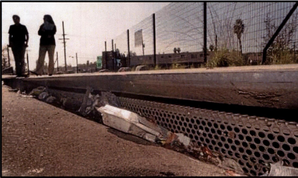
Image Credit: An automatic retractable screen prevents trash from entering a storm drain in Valley Glen, CA. (File photo by Dean Musgrove/Staff Photographer, Los Angeles Daily News) accessed: https://www.dailynews.com/2017/04/21/capturing-stormwater-and-planning-for-californias-future-bob-hertzberg/
