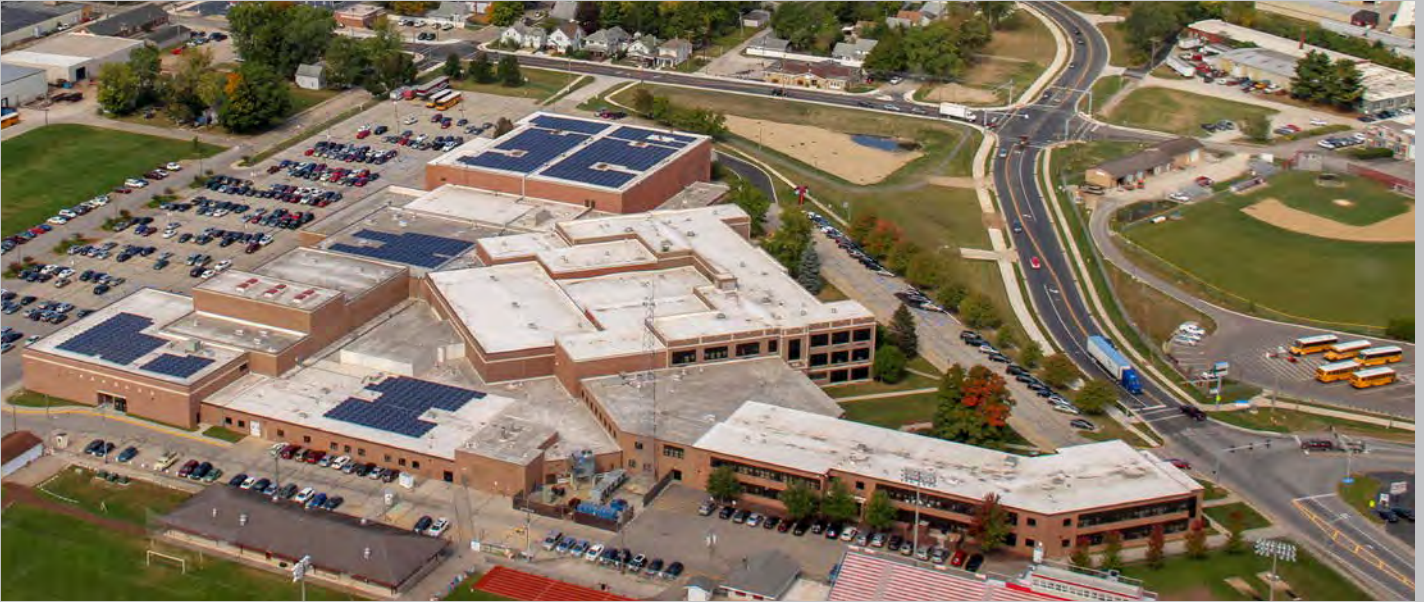
SOLAR PANELS AT GOSHEN HIGH SCHOOL
