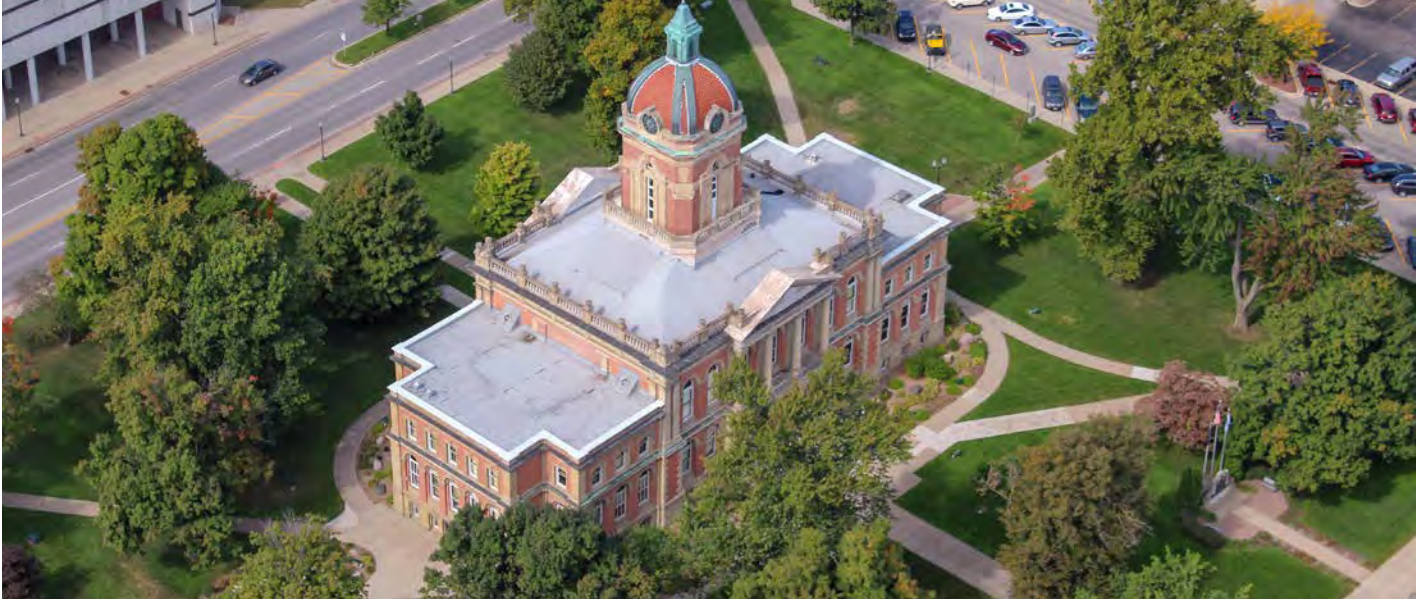
ELKHART COUNTY COURTHOUSE, DOWNTOWN GOSHEN
