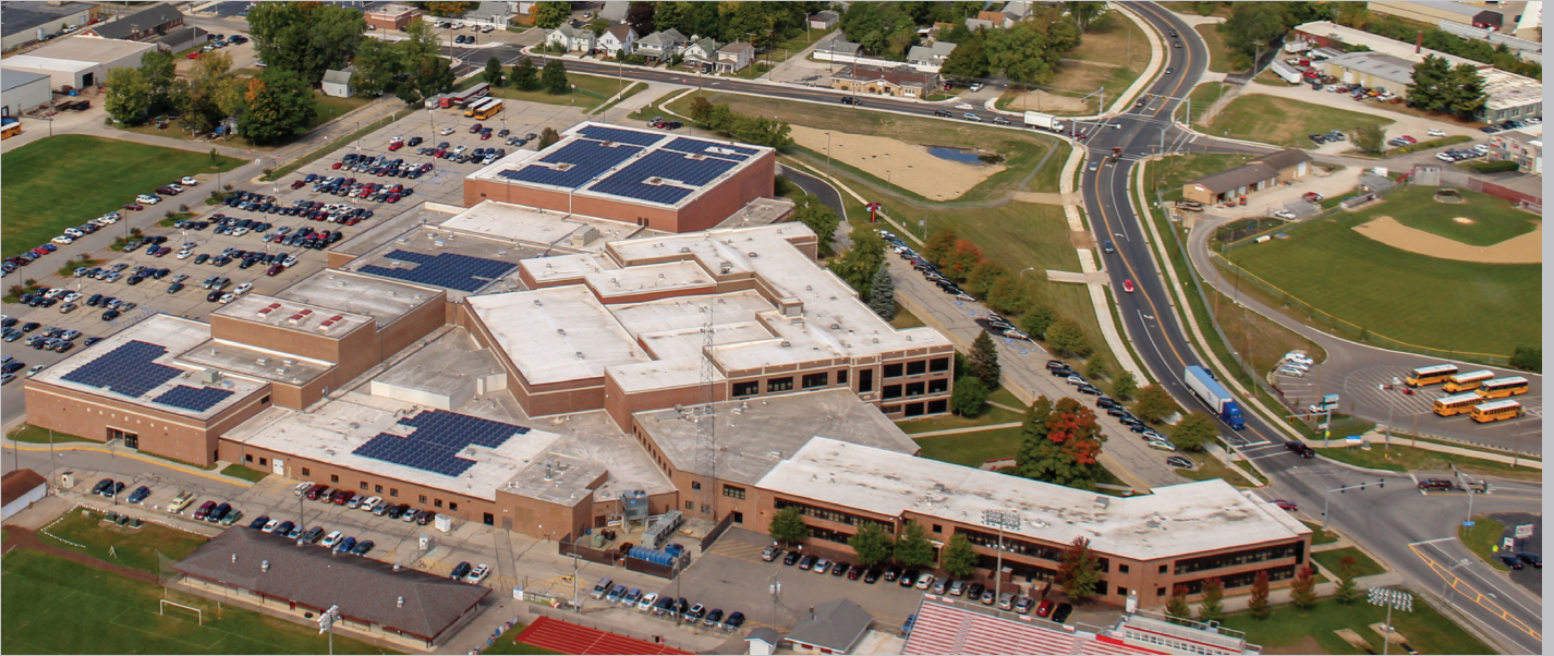
SOLAR PANELS AT GOSHEN HIGH SCHOOL
