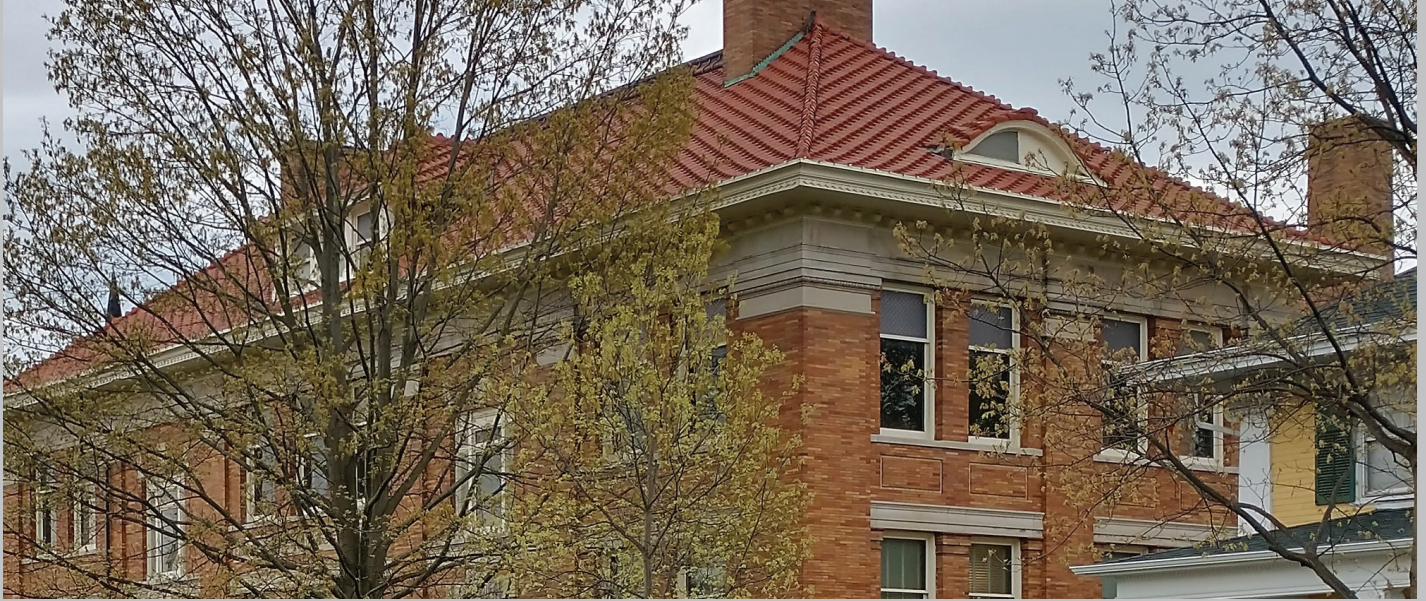
CITY ANNEX BUILDING
