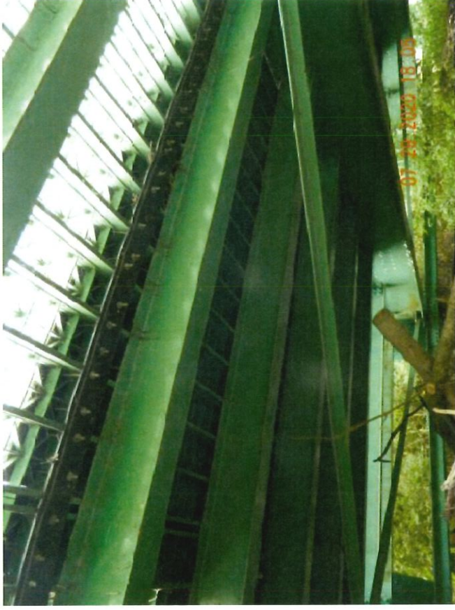
TYPICAL UNDERSIDE OF BRIDGE
