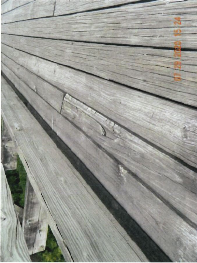
CHECKING OF TIMBER DECK
