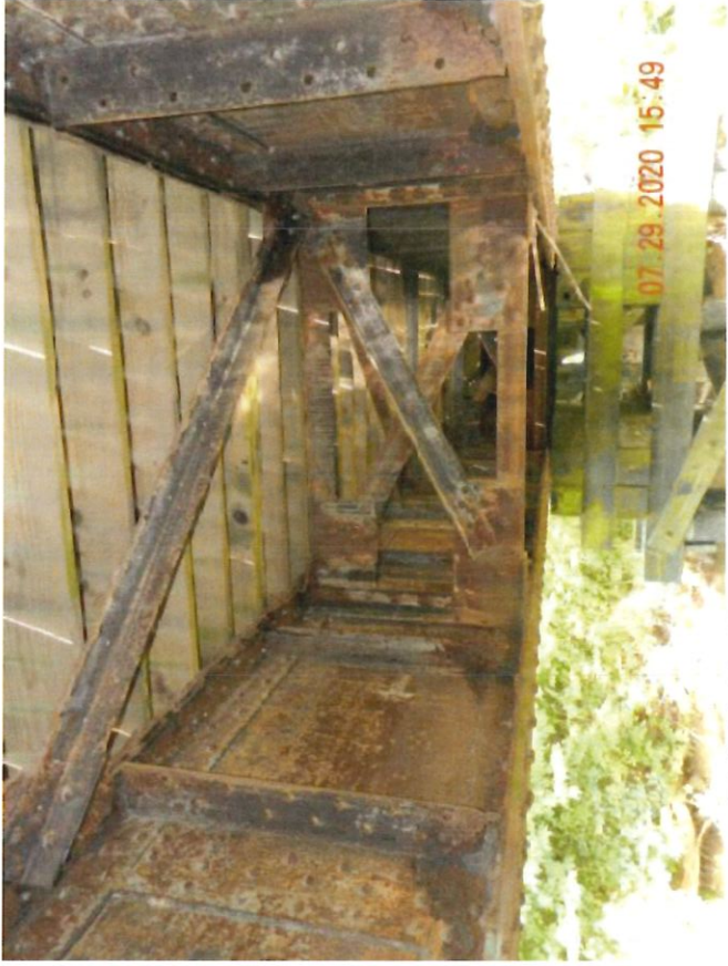
TYPICAL UNDERSIDE OF MAIN SPAN
