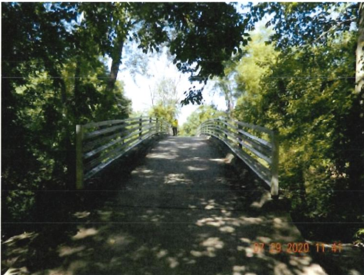
SECTION LOOKING WEST
