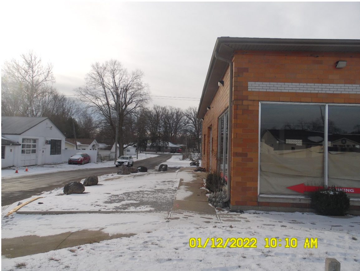
Looking south along east wall of building
