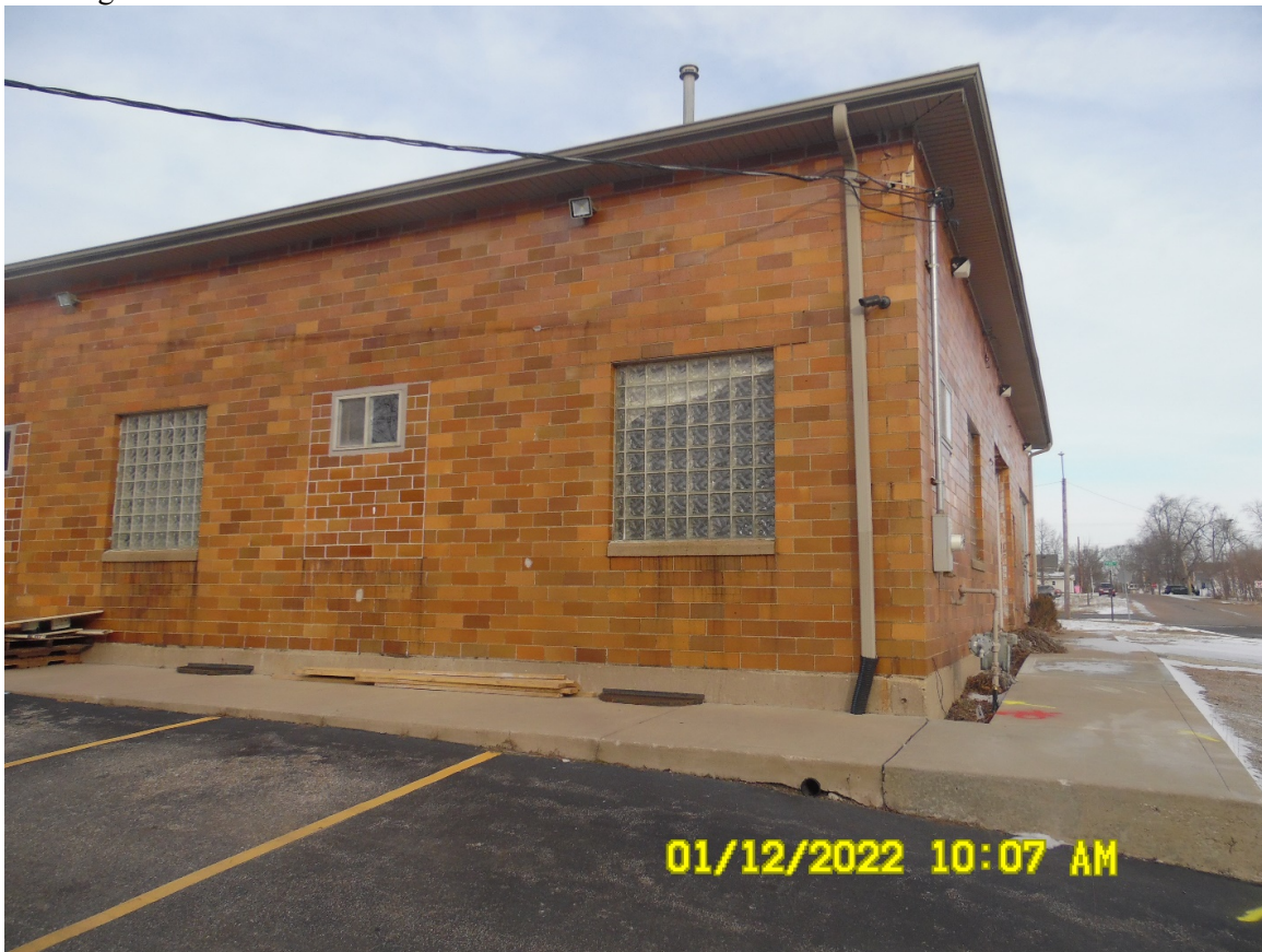
Looking north-northwest at proposed location of freezer
