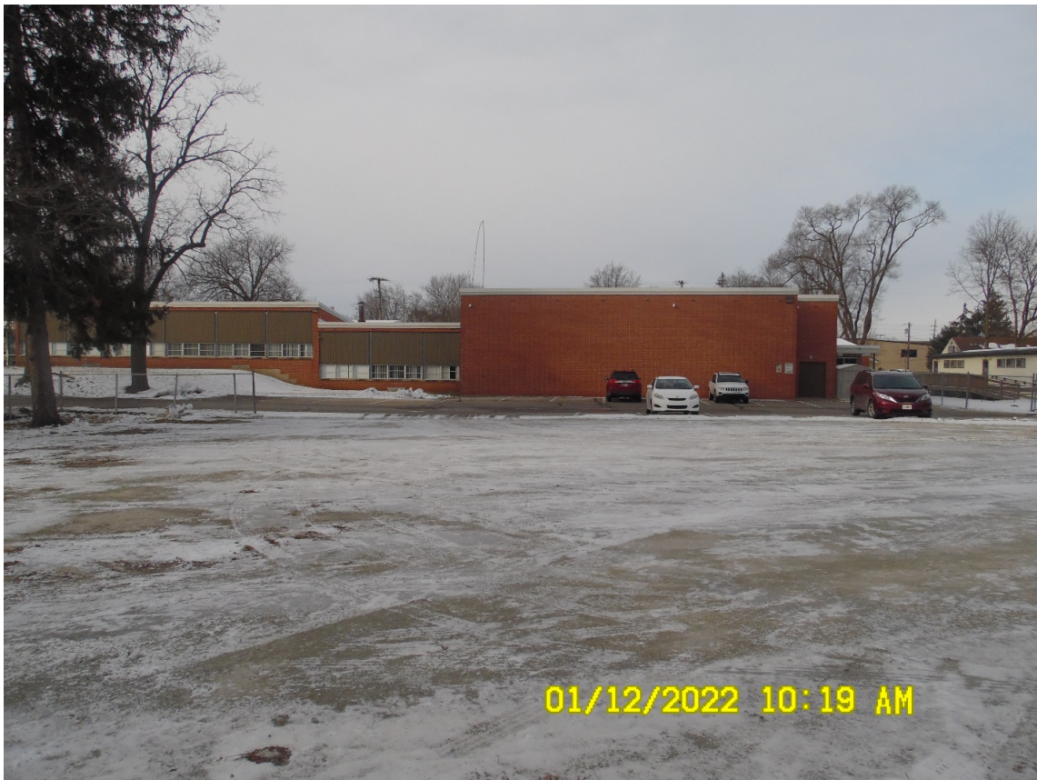
Looking west at available parking on east side of building
