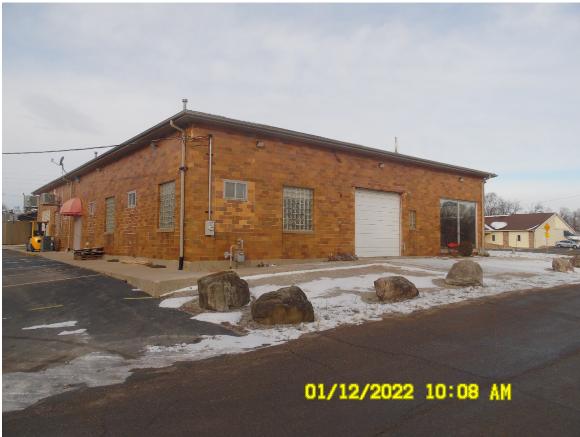
Looking northwest from Harrison Street
