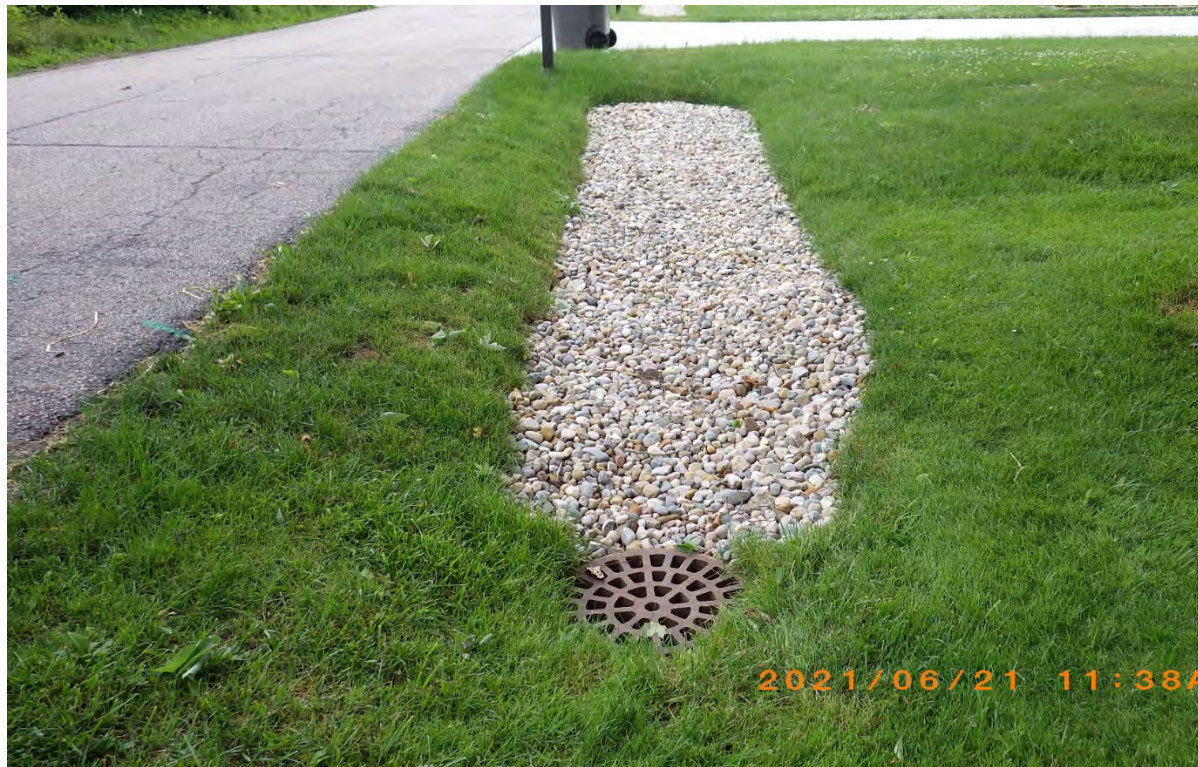
Carter Road Drainage Swale Improvement
