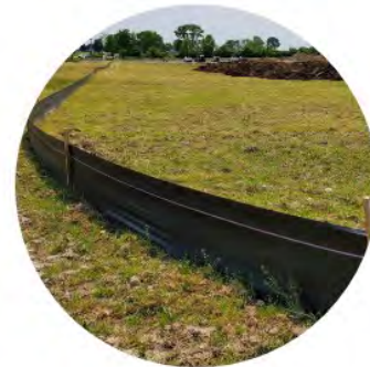
Construction Site Stormwater Run-off Management*
