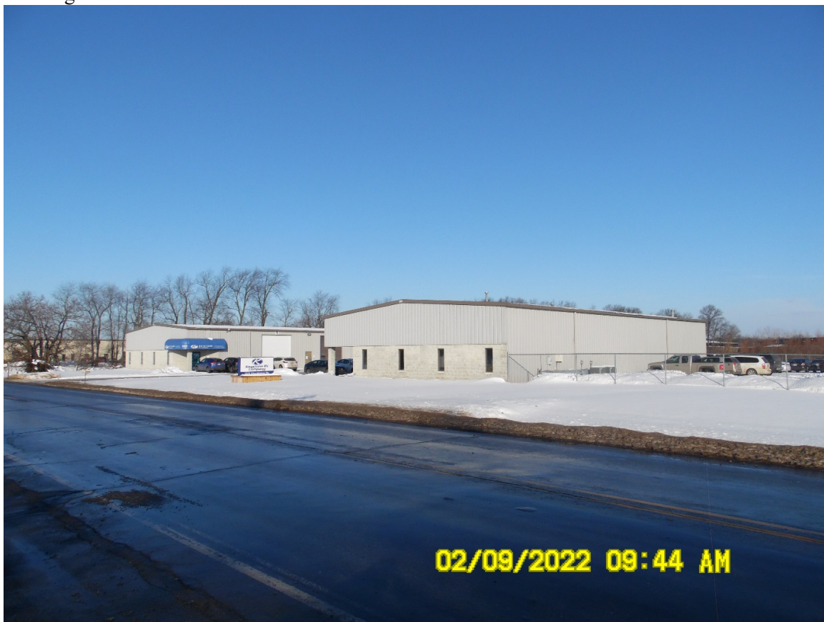
Looking northwest from Eisenhower Drive North
