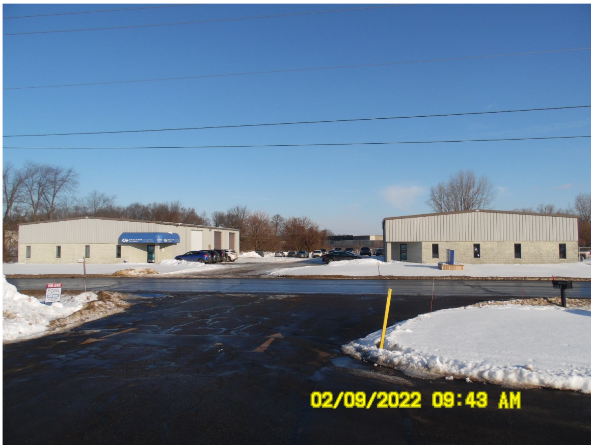
Looking north across Eisenhower Drive North.
