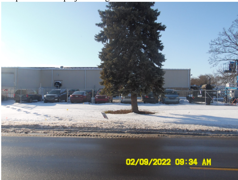
Looking south at proposed location of new access drive to loading dock
