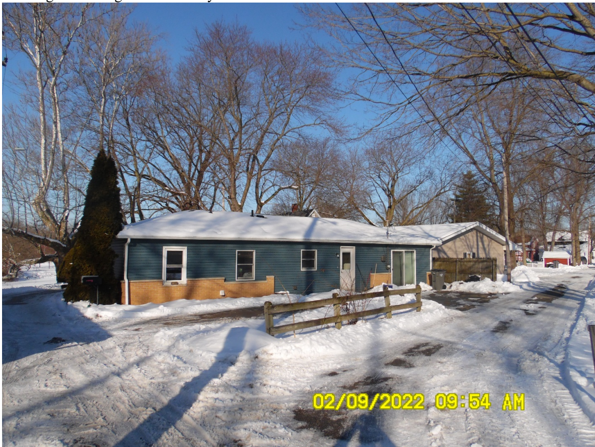
Looking northwest at rear of home and location of proposed addition
