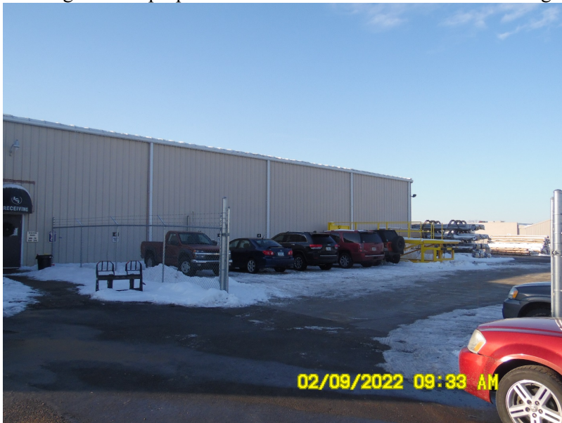
Looking southwest at portion of building where loading dock will be installed.
