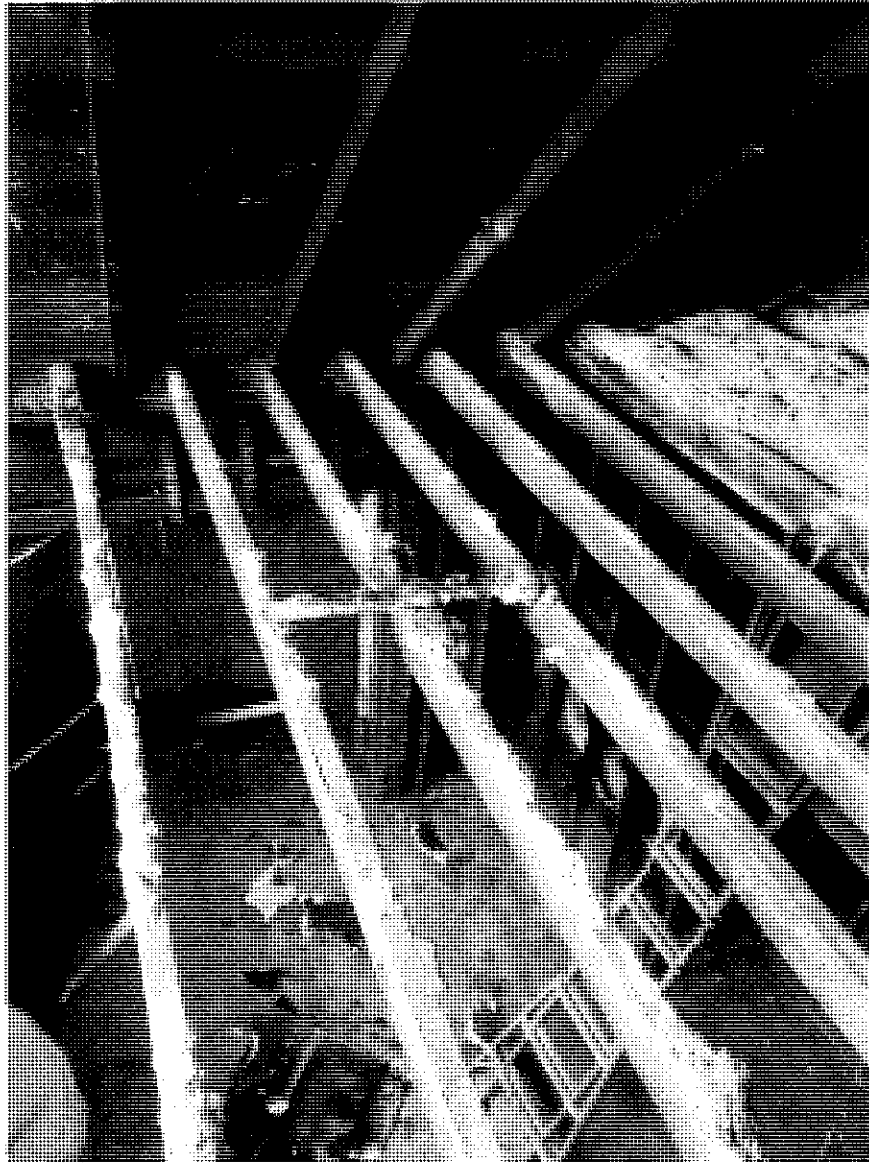
Ceiling Joist – not damaged
