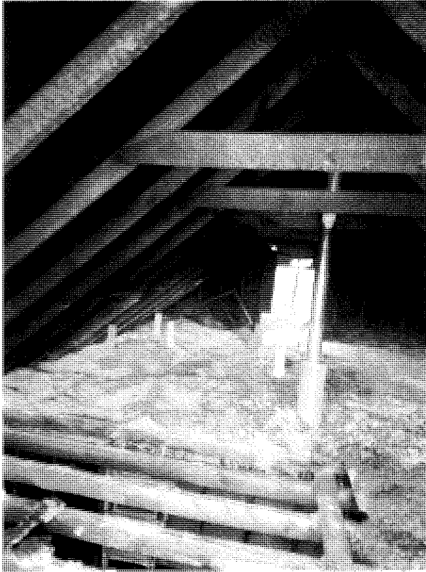
Back half more smoke damage than structural
