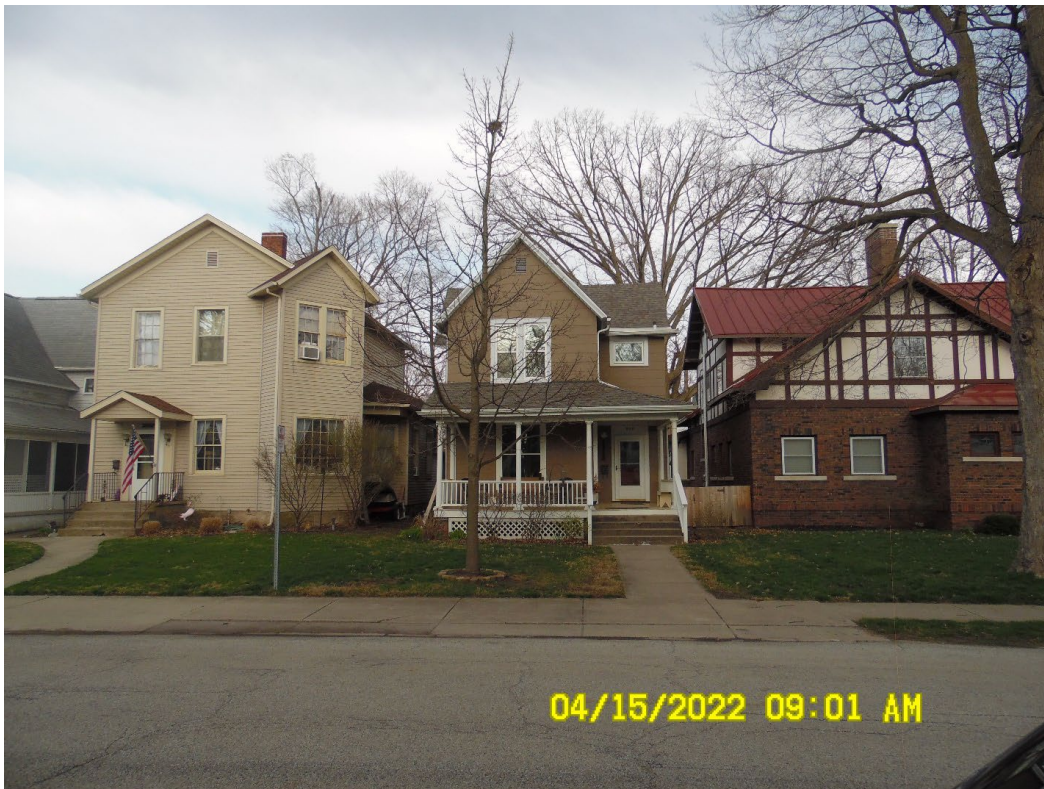
Looking west across S 6 th Street at front of home
