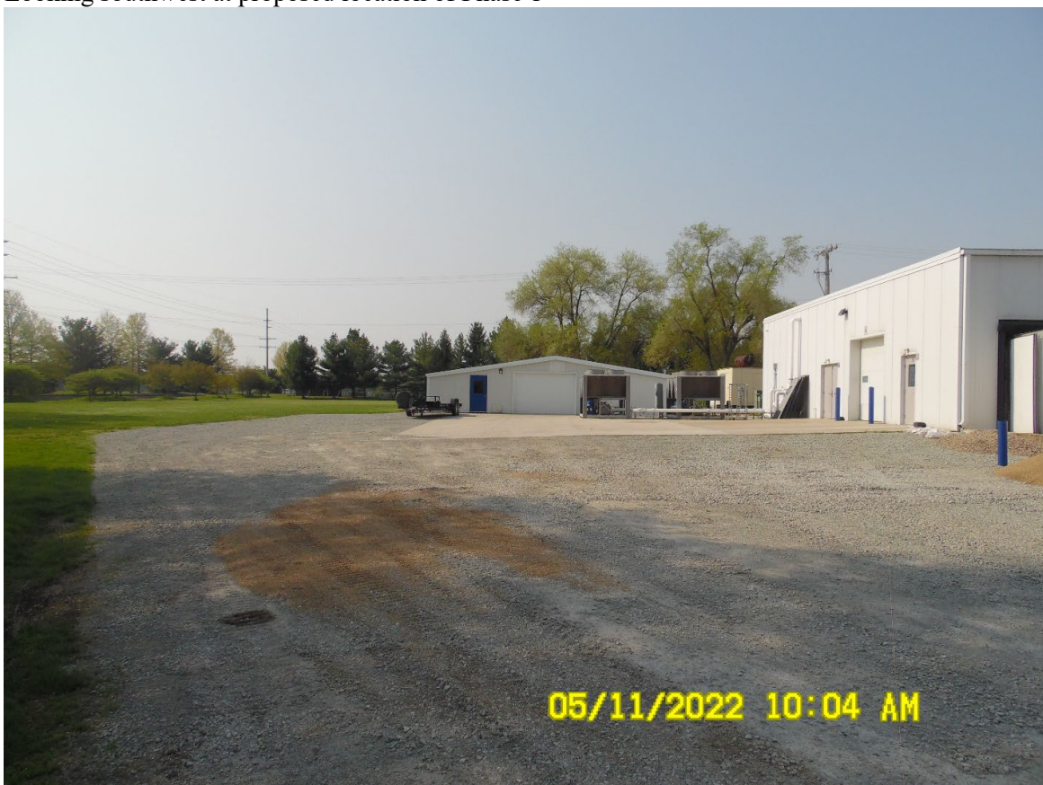
Looking south at proposed location of Phase 3 with detached accessory building in background
