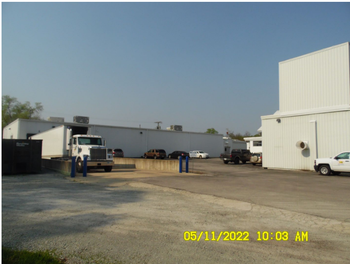
Looking southwest at proposed location of Phase 1
