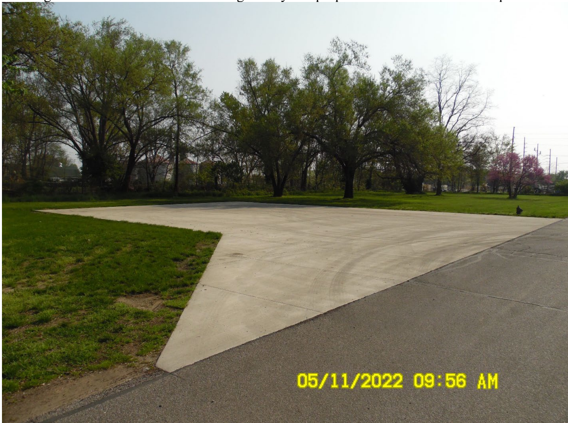
Looking northeast at unapproved concrete maneuvering area
