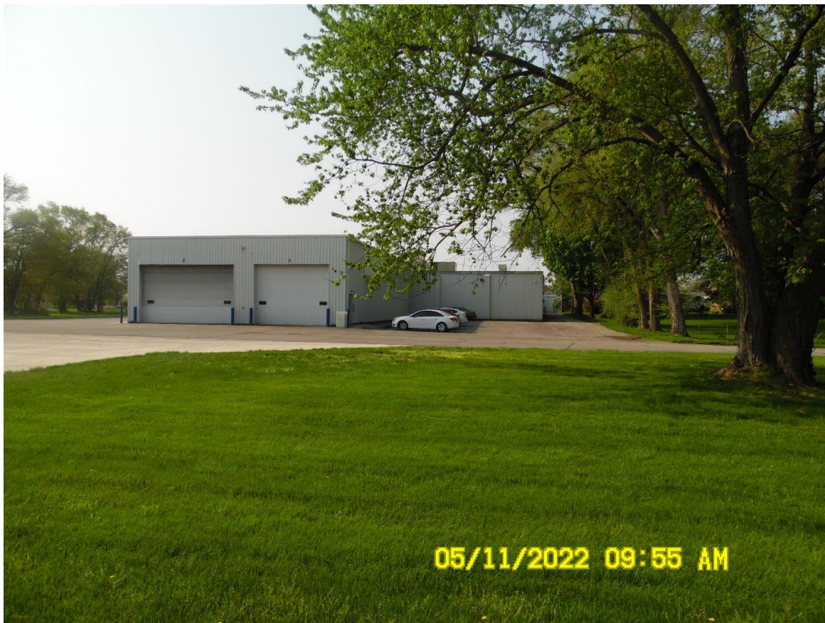
Looking south at north end of the existing facility and proposed location of Phase 2 expansion
