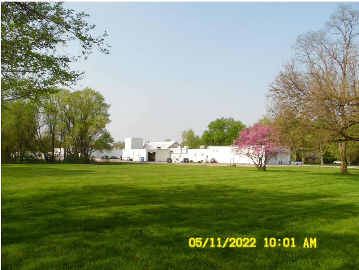
Looking southwest at proposed location of Phase 4
