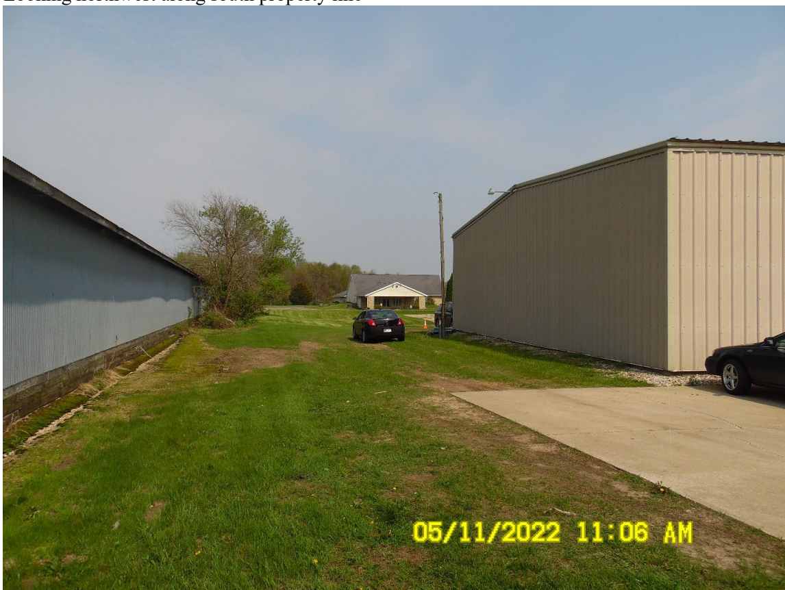
Looking at south end of west building
