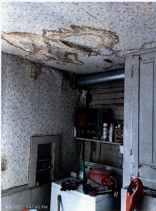
Water damage from previous roof leak
