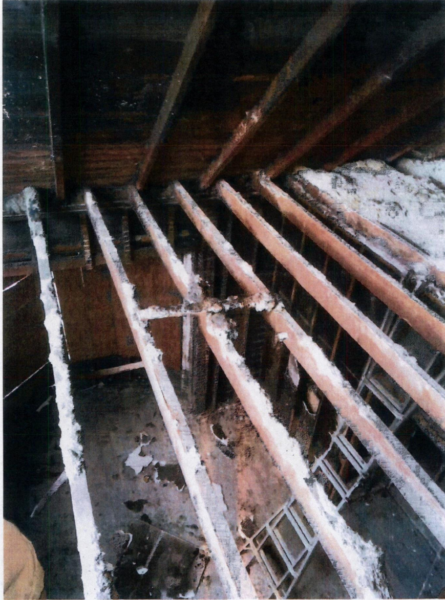
Ceiling Joist – not damaged
