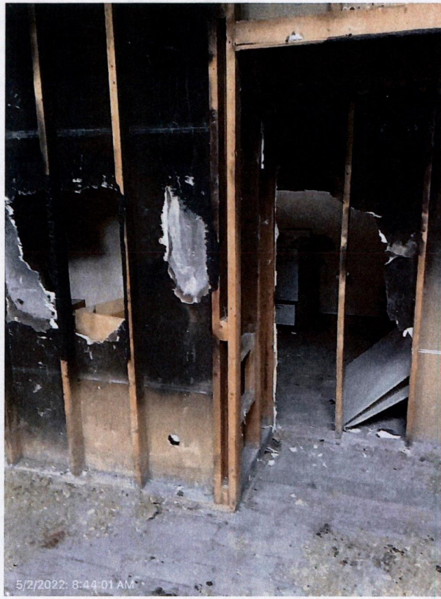
Five damaged drywall and beams
