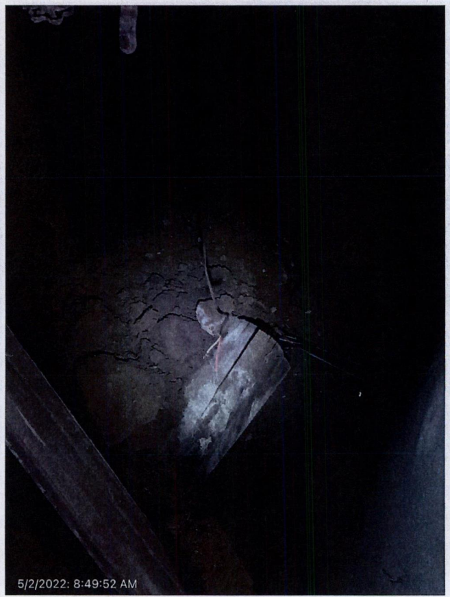
exposed wires and wash out accumulation from foundation
