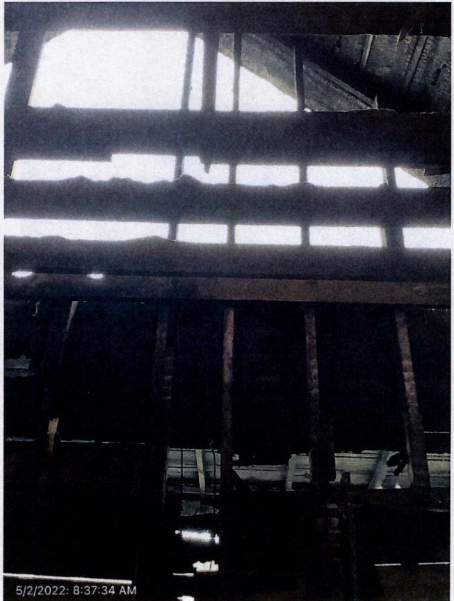
Front wall and attic from inside
