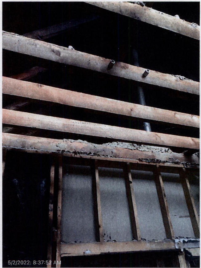
Looking into attic from front room
