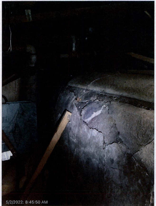
Basement wall cracking
