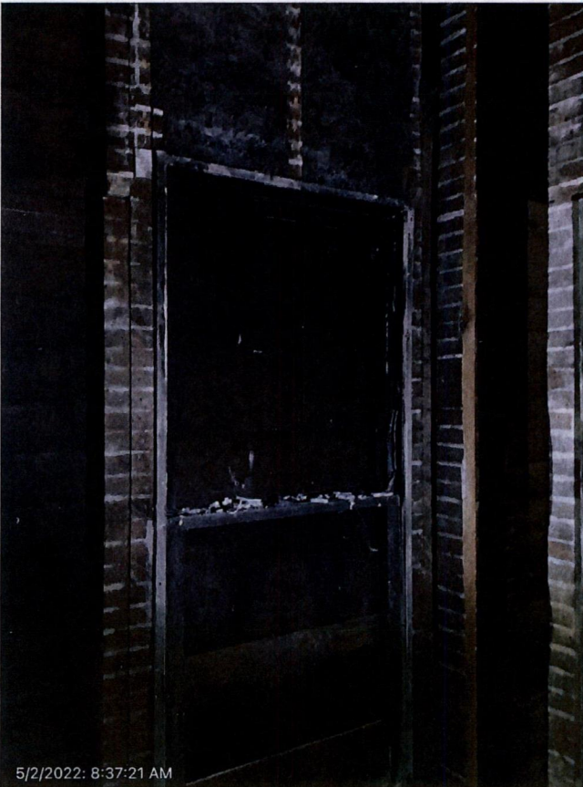
Burnt out window frame
