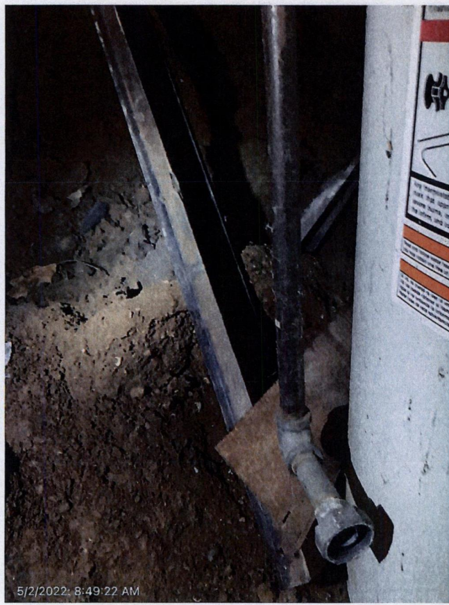
more washout from basement wall collapsing
