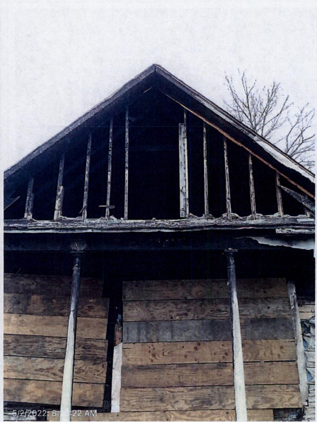
Front wall & attic fire damaged
