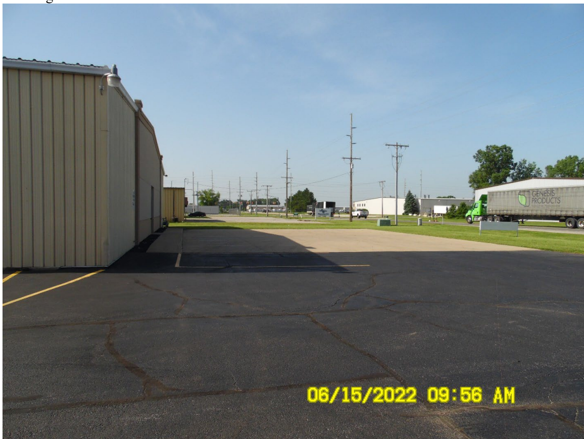
Looking south across front of south building
