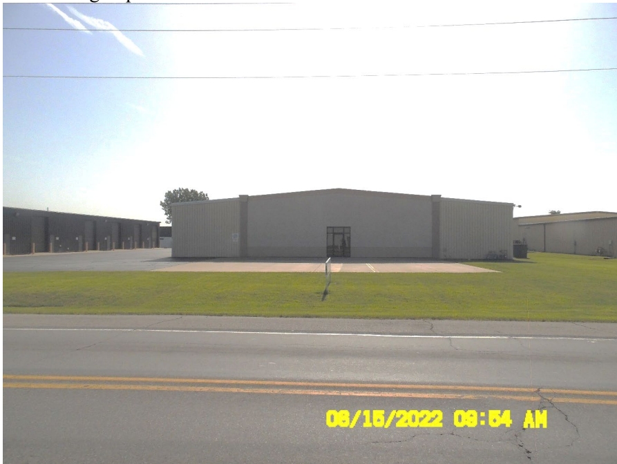
Looking east across Dierdorff Road
