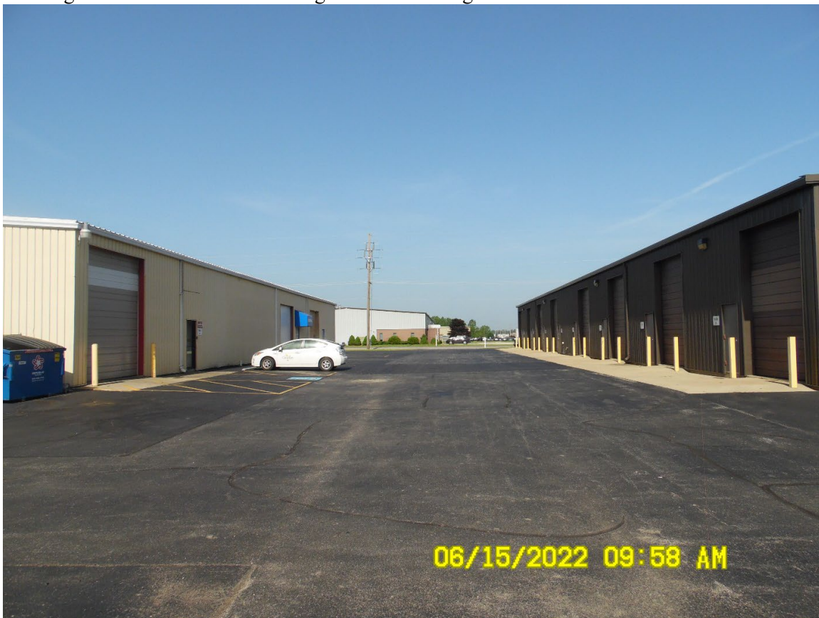
Looking west between north and south buildings
