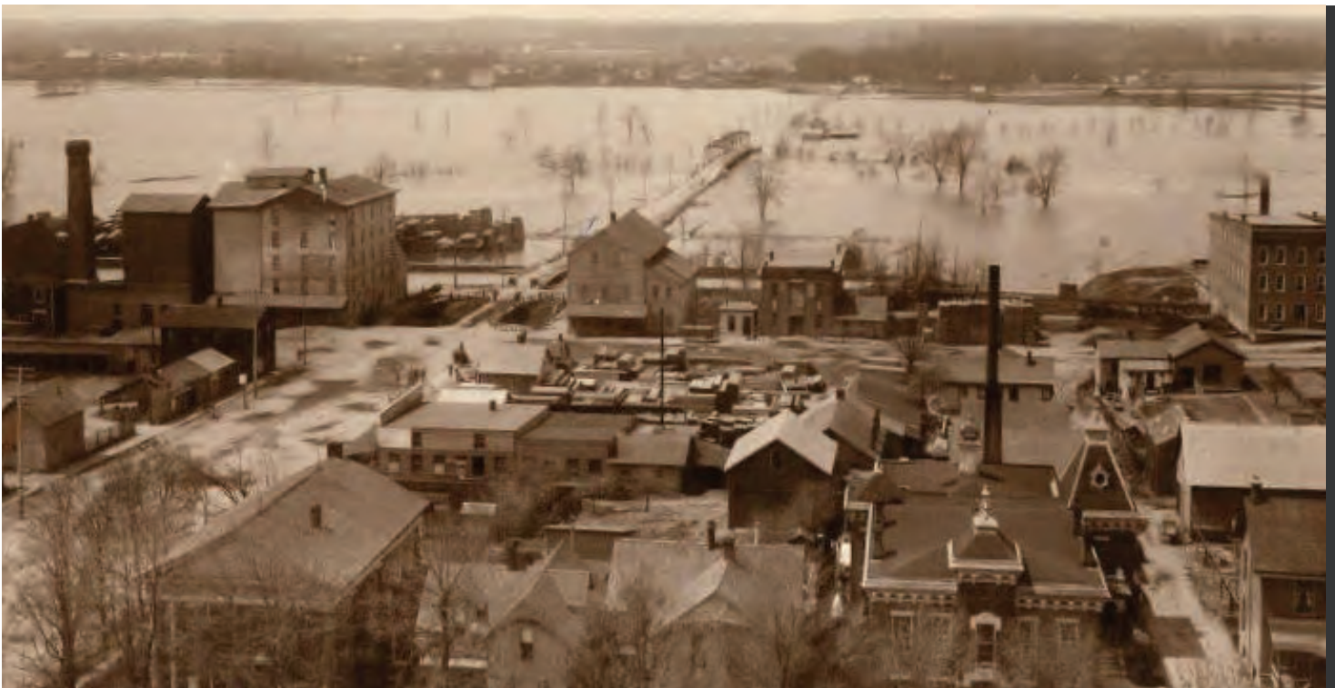
1892 – View of Lincoln Ave. bridge from County Courthouse
