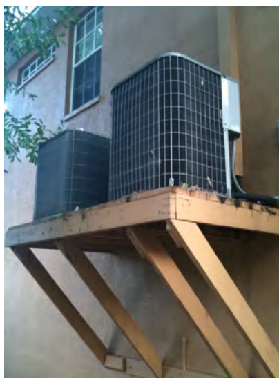
Figure 6-9: Example of Compliance with Flood Ordinance Requirements
