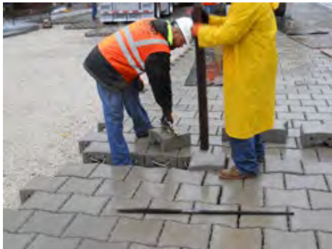
Figure 5-1: Installation of Permeable Paver System in Goshen
