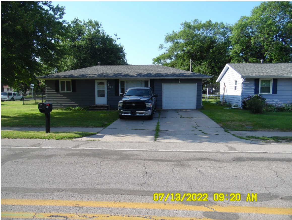
Looking south from Plymouth Avenue at existing one-stall garage and open parking space
