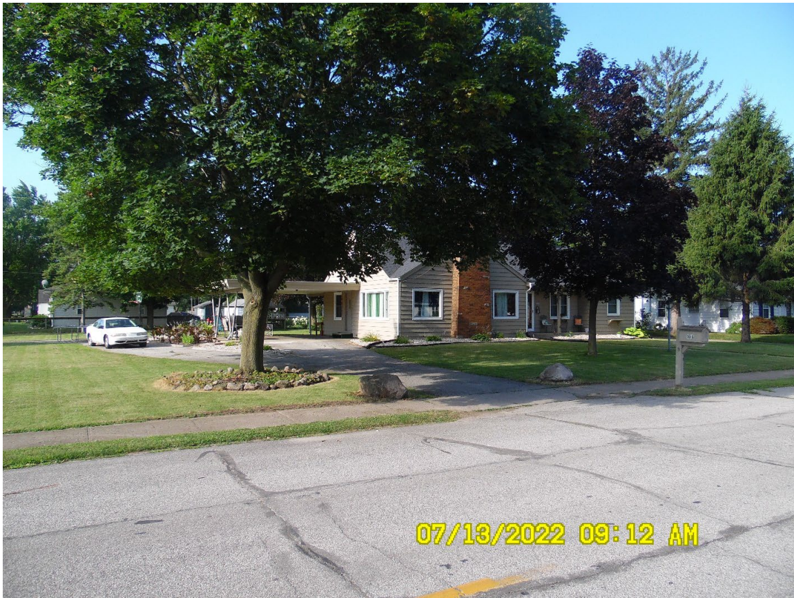
Looking southwest from Reynolds Street at 908 E Reynolds
