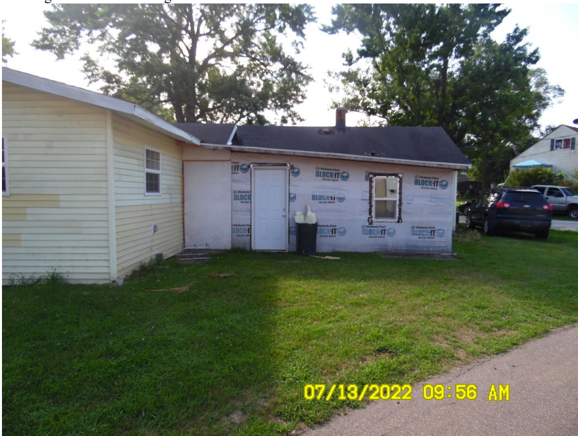
Looking southeast from Westfield Avenue at location of proposed garage rebuild
