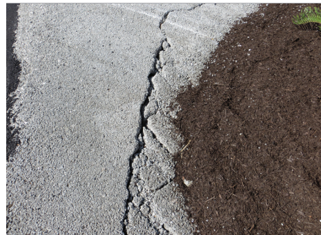
7 CRACKING-STRUCTURAL
