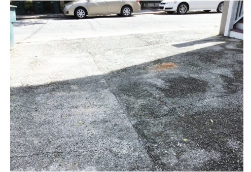
7 CRACKING-STRUCTURAL
