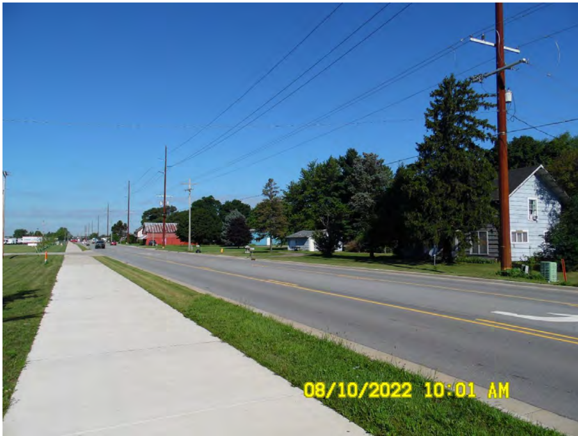
Looking northwest along Kercher Road
