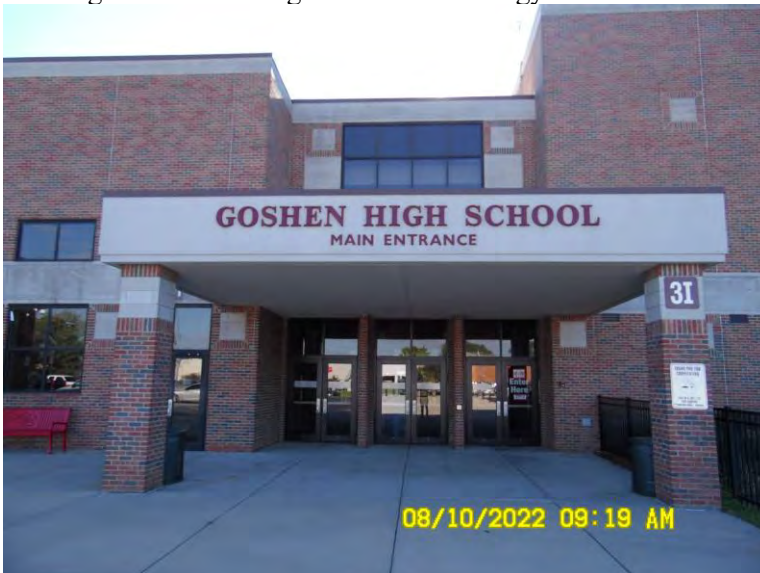
Looking east at wall sign on main entrance canopy
