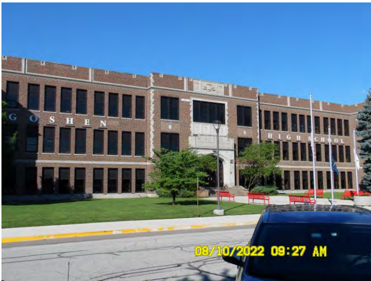
Looking west at wall sign on east side of building
