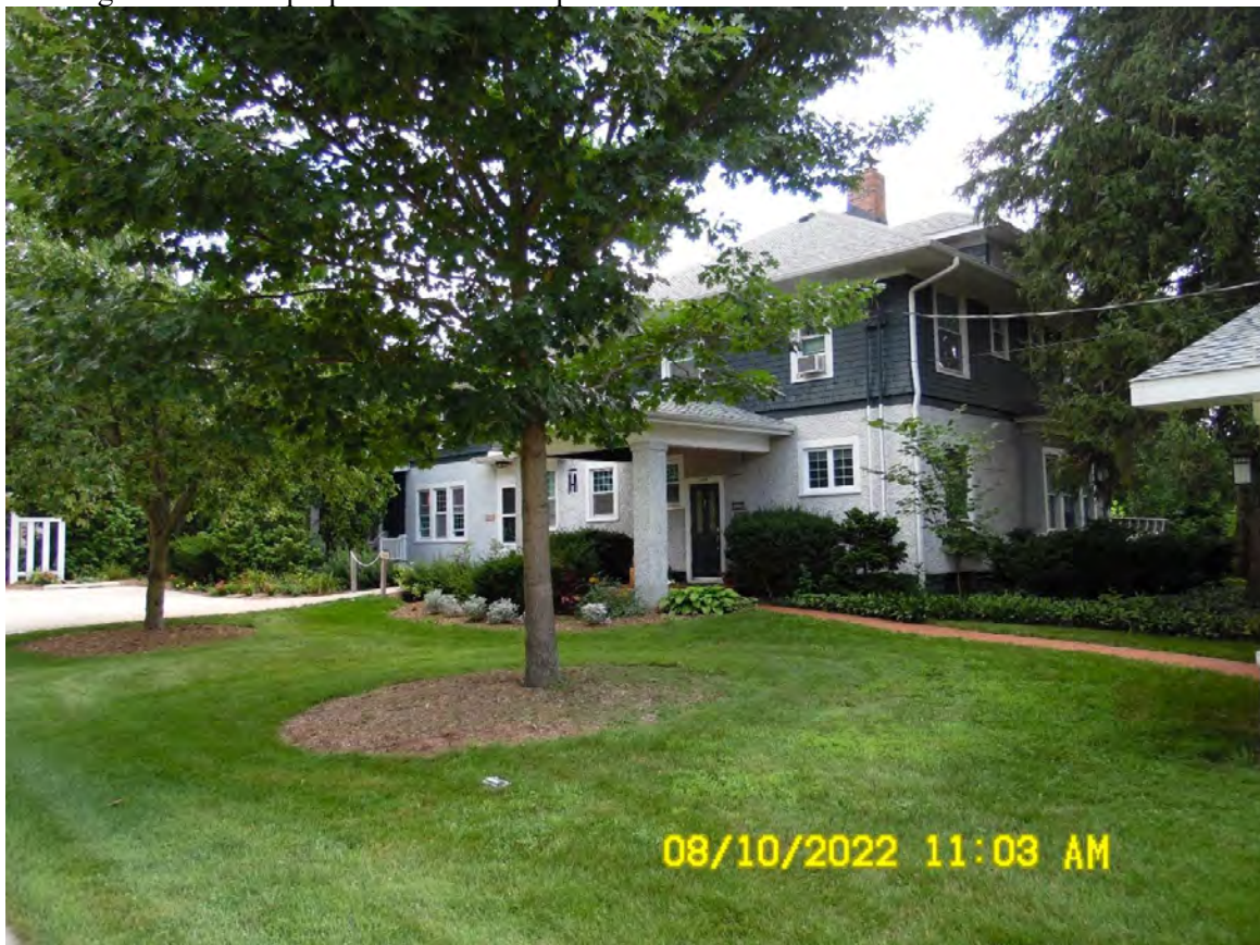
Looking northeast at residence and retreat center building
