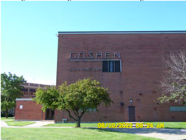
Looking south at wall sign on north side of gym
