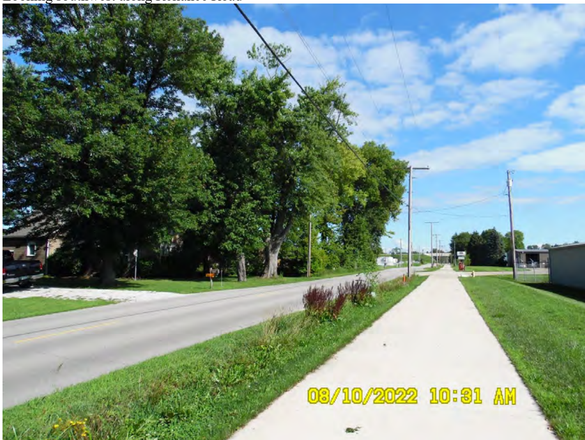
Looking north-northwest along Reliance Road
