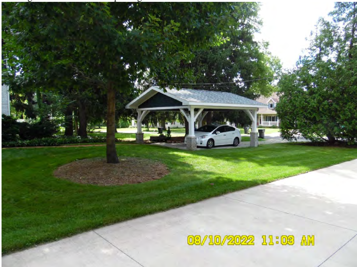
Looking southeast at 2-stall carport that serves the residential use
