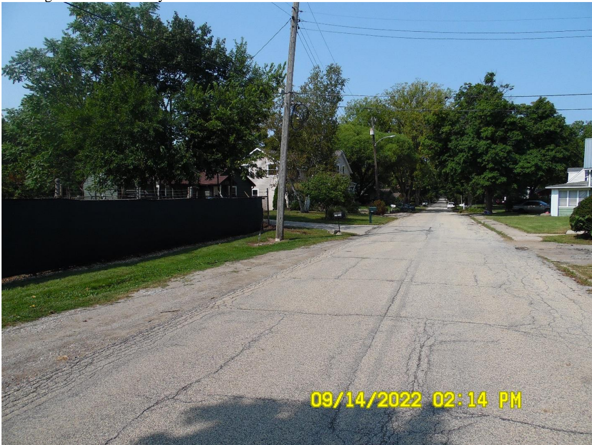
Looking north-northwest along Wilson Avenue
