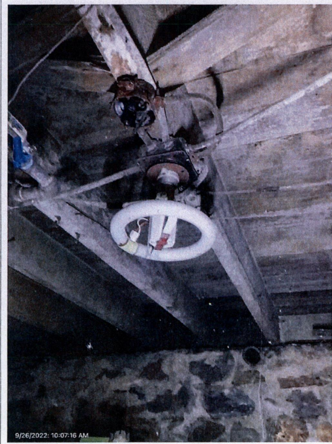
Electrical wiring exposed
