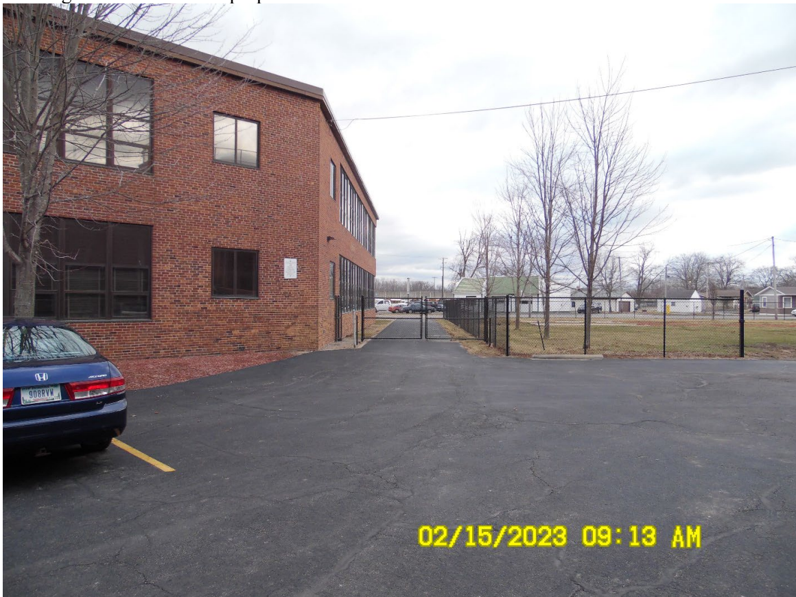
Looking northeast at the location of the eastern-most entrance
