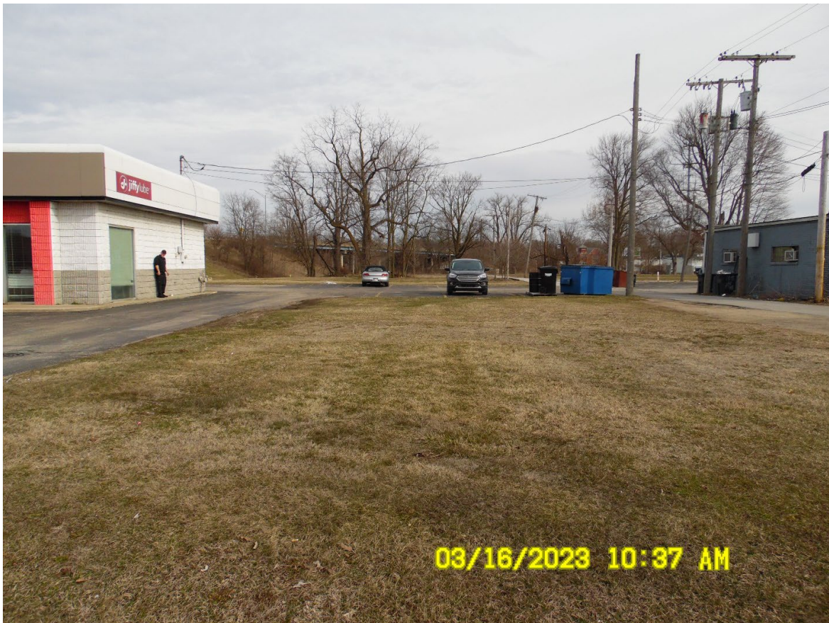
Looking north at the proposed location of the building addition and parking and driving aisle expansion
