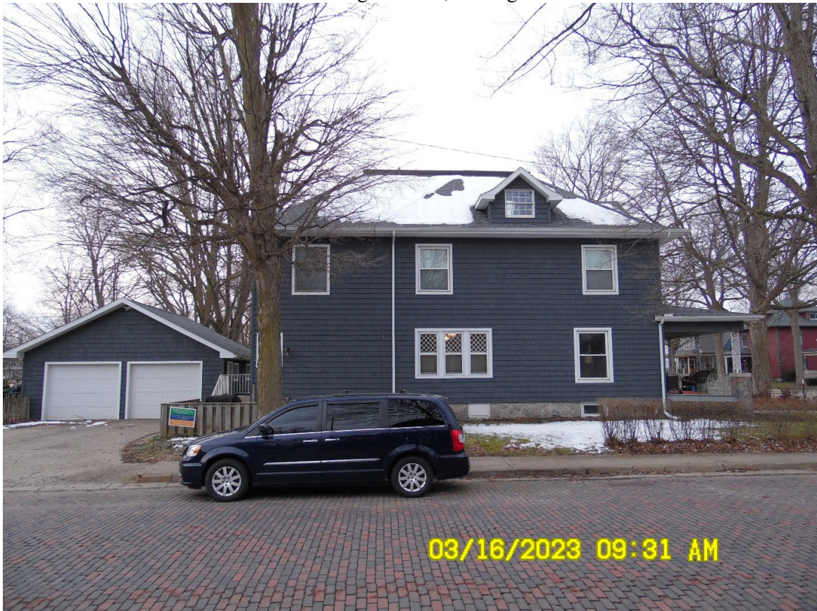
From Douglas Street, looking south
