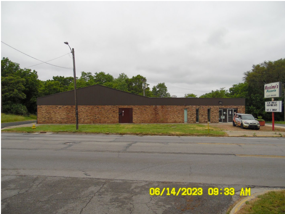
Looking west across Main Street
