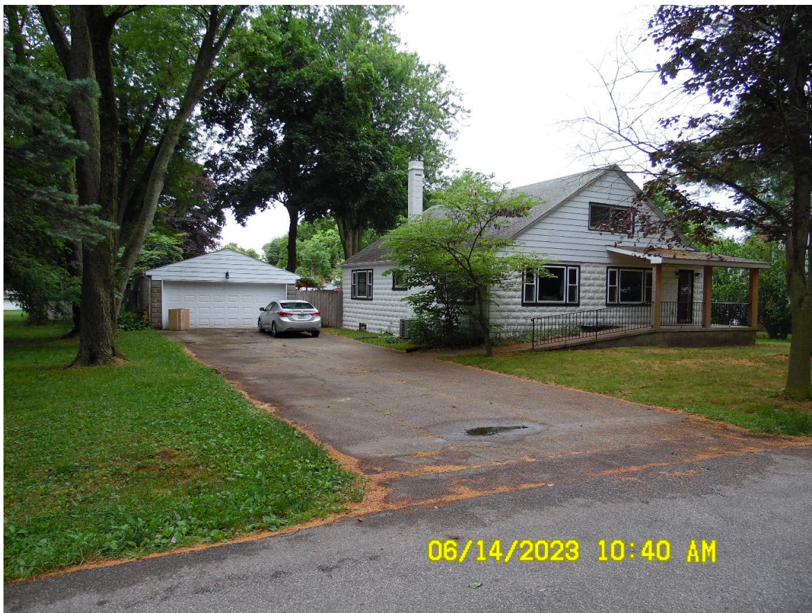
Looking northwest from Winter Avenue
