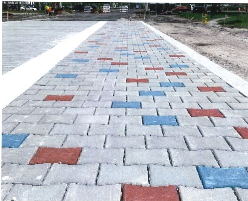
Optional Multi-color Pave Drain Installation
