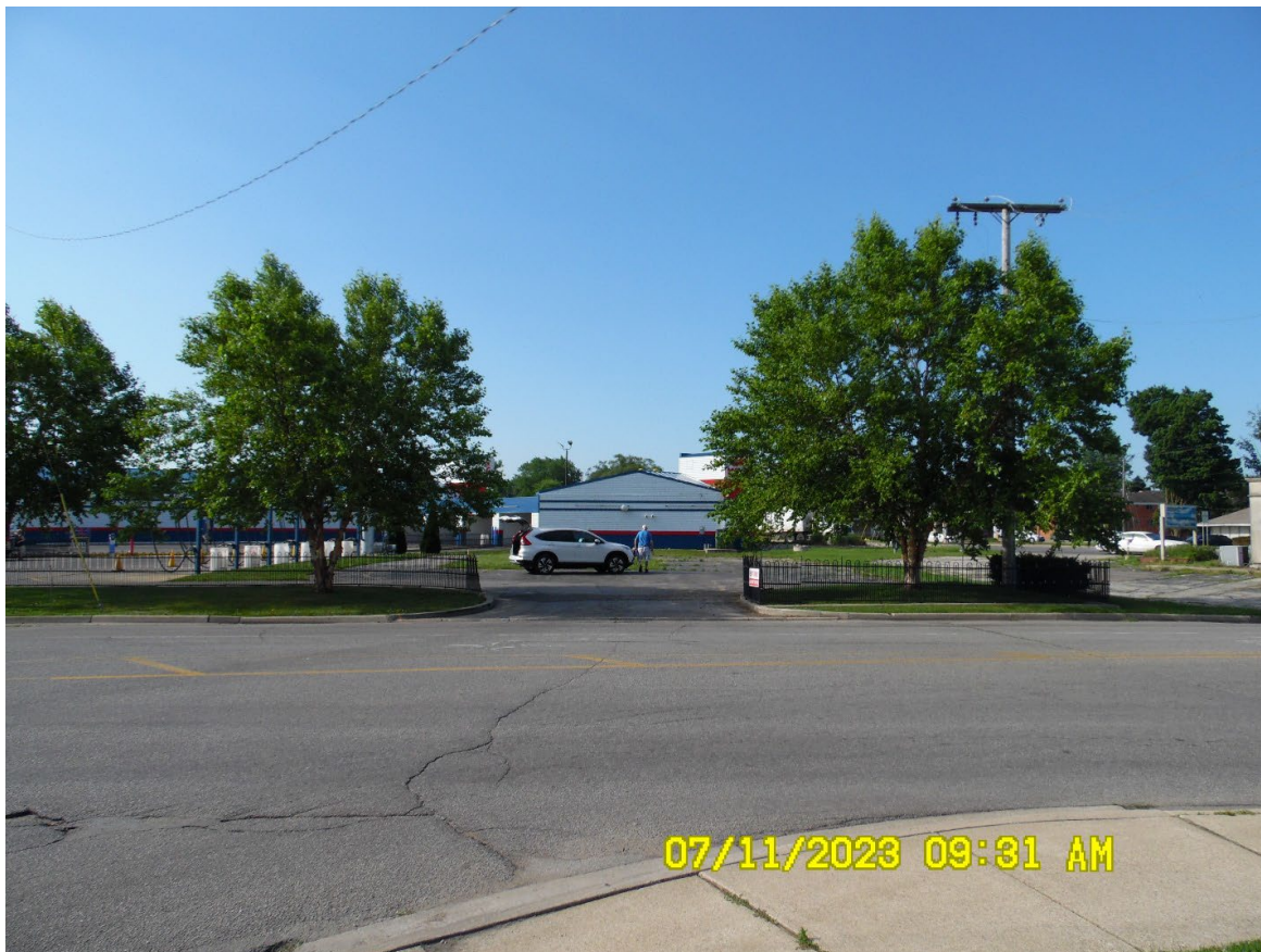
Looking south across Bashor Road
