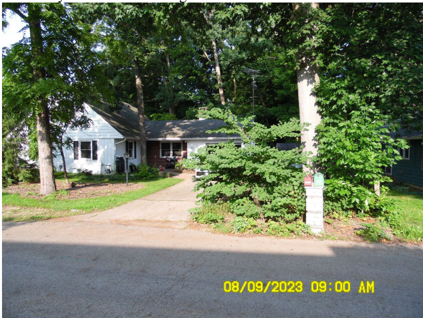
From Mayflower drive looking west along the north property line
