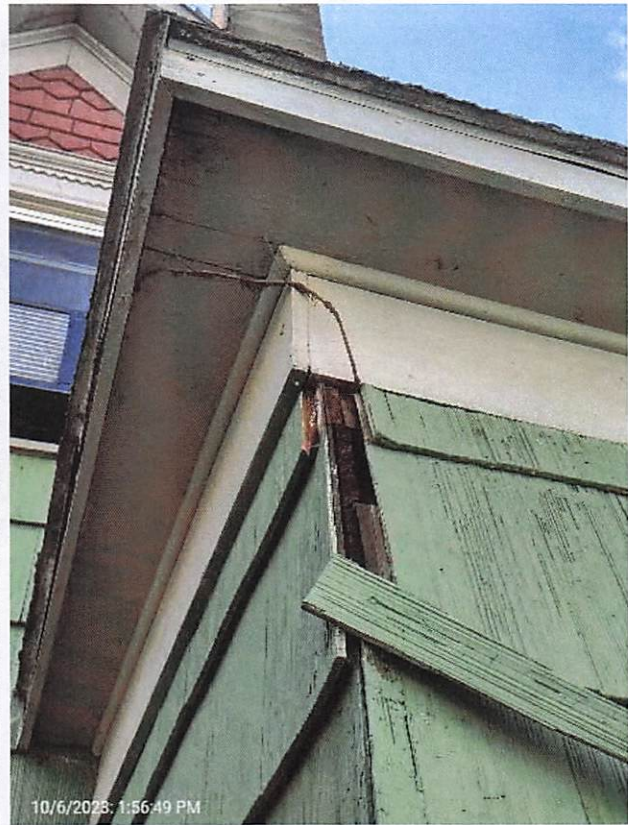
Loose siding at rear of property.
