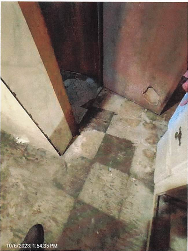
10/6/2023: 1:54:35 PM Wood flooring in bathroom.
