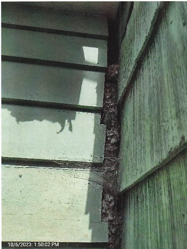
Gap in wood siding at rear of property.
