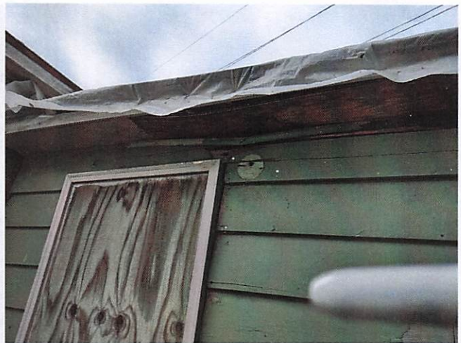
Plastic covering roof at rear of property.
