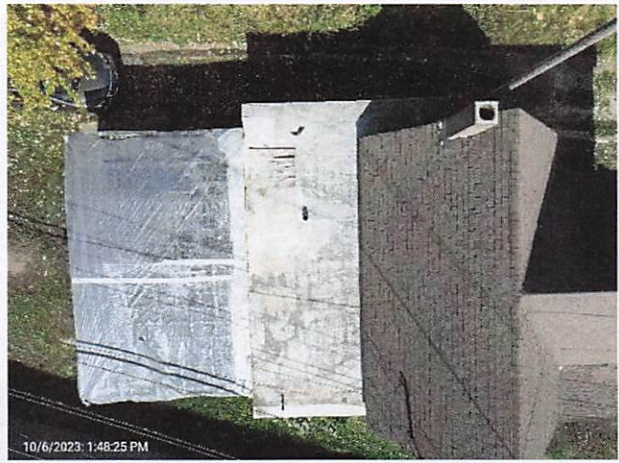
Overhead view of roof at rear of property.
