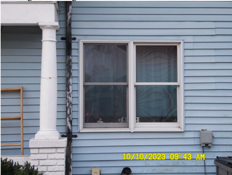
Looking south at proposed window location for 2 illuminated signs
