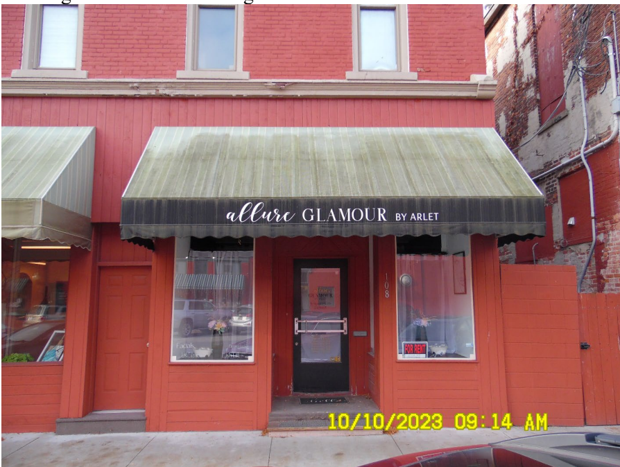
Looking west at 108 E Washington Street
