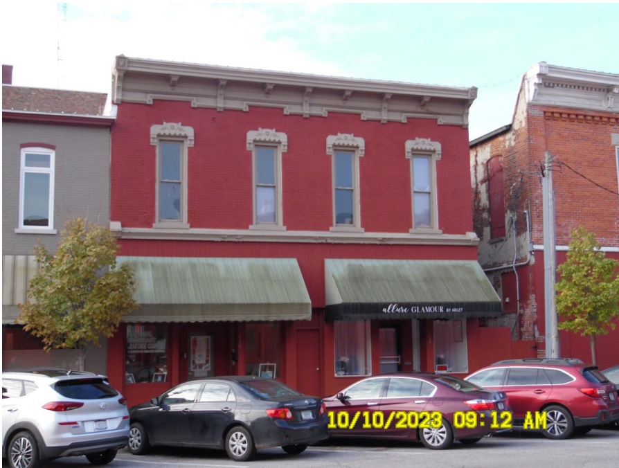
Looking south across Washington Street
