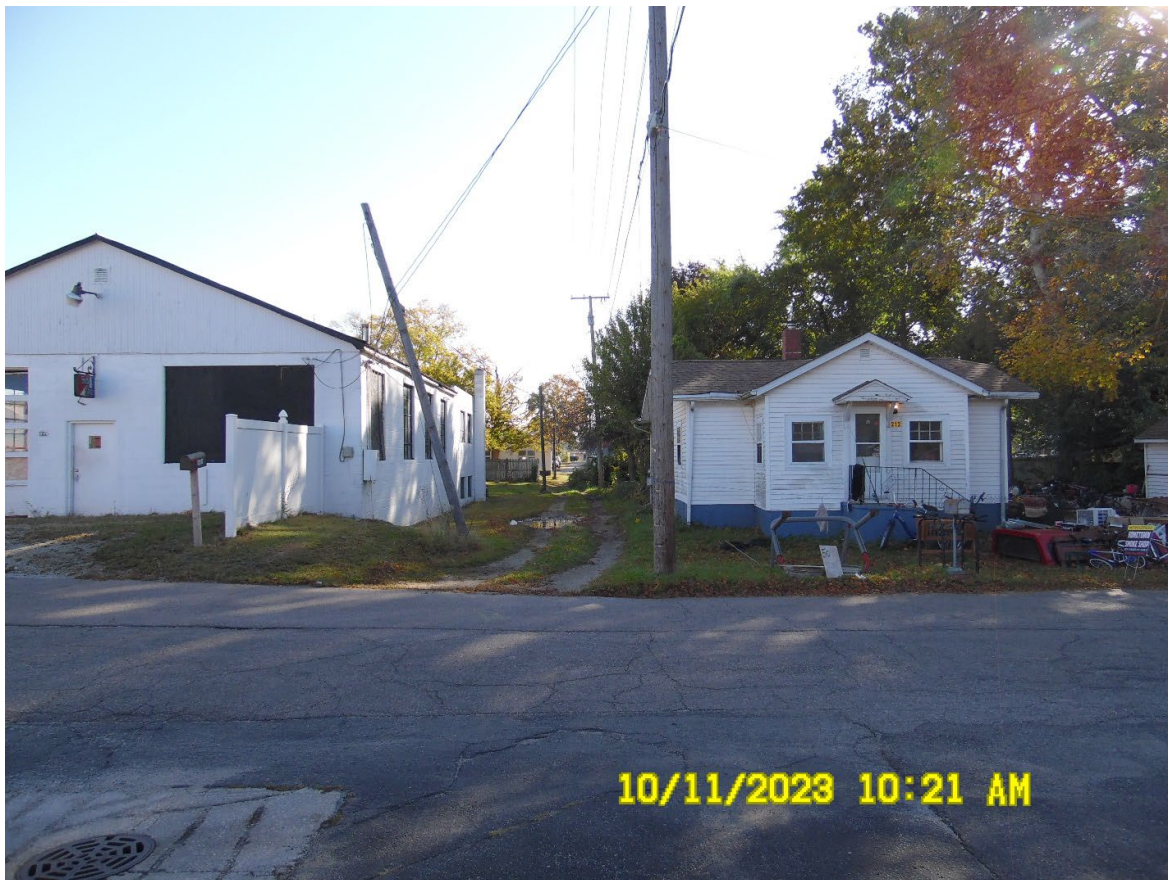
Looking east across Harrison Street at south property line and vacated alley (utility easement)
