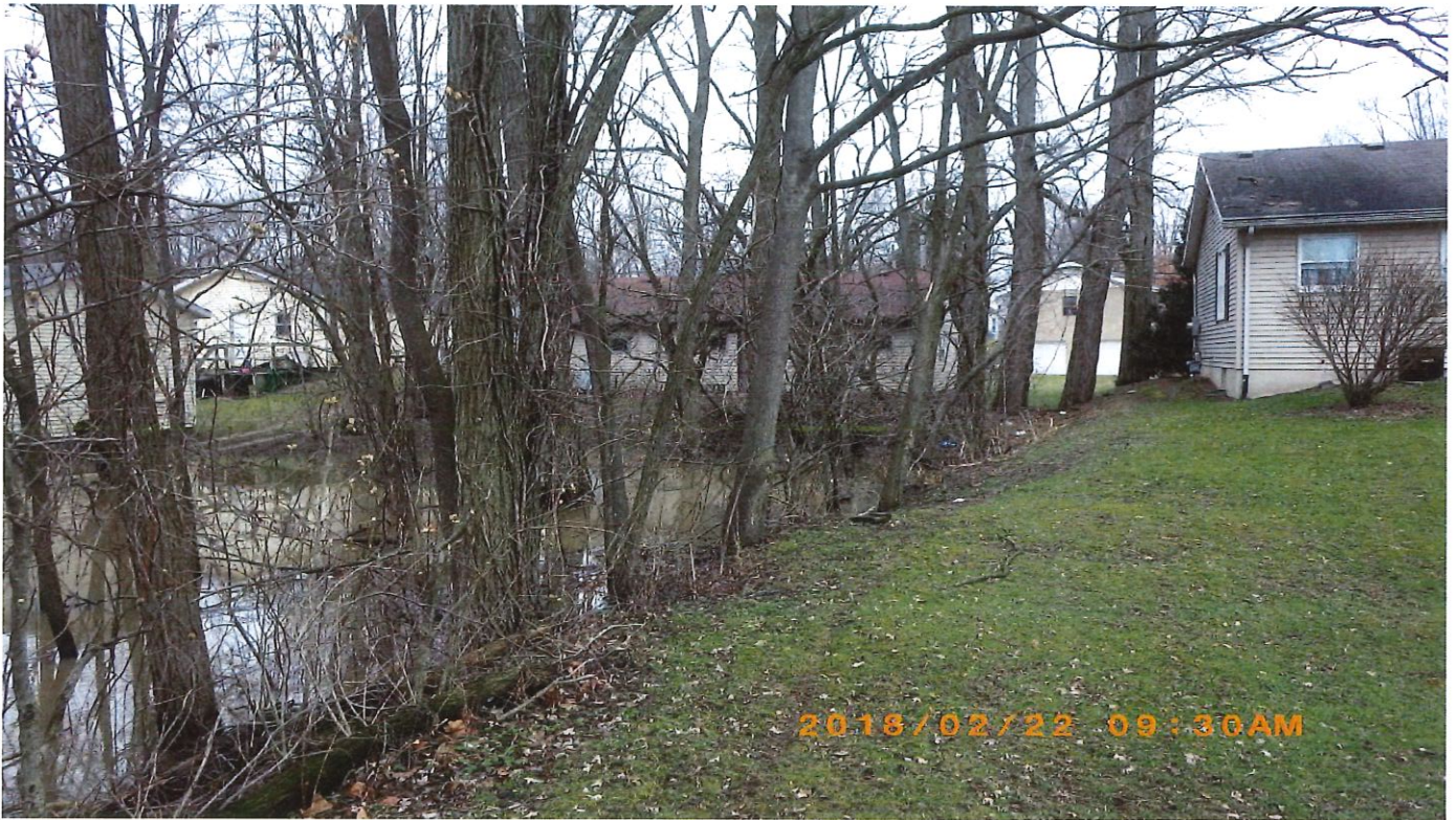
Looking west; 302 S Indiana Ave is on the right, 304 S Indiana Ave is in the middle, and 308 S Indiana Ave is on the left of the picture. (Image Date: February 22, 2018, Photo credit: Jason Kauffman)
