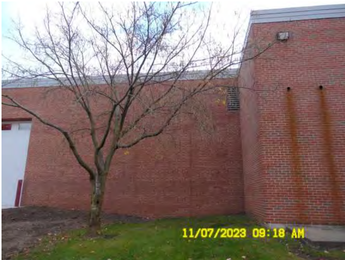
Looking east at proposed dust collector location
