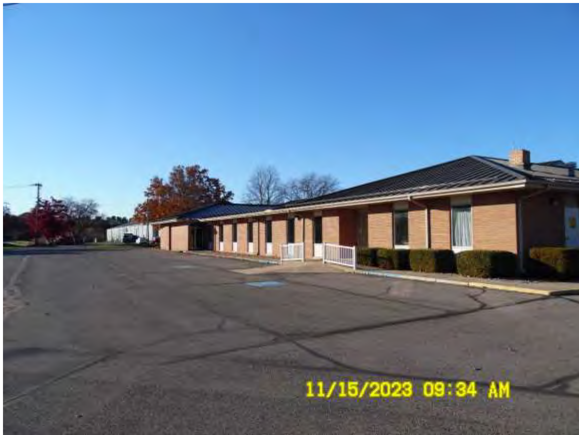
Looking southwest at the east side of the building
