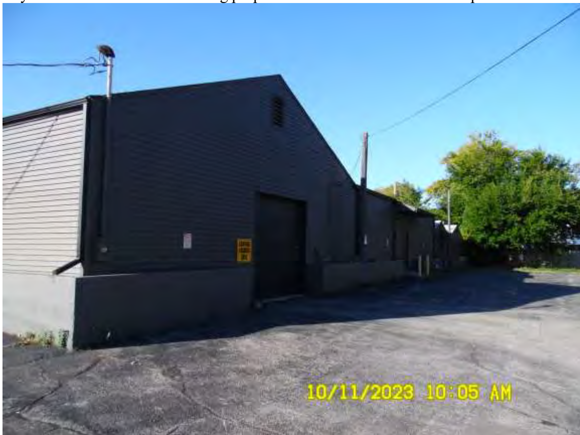
Exterior view of bay door on northeast corner of building
