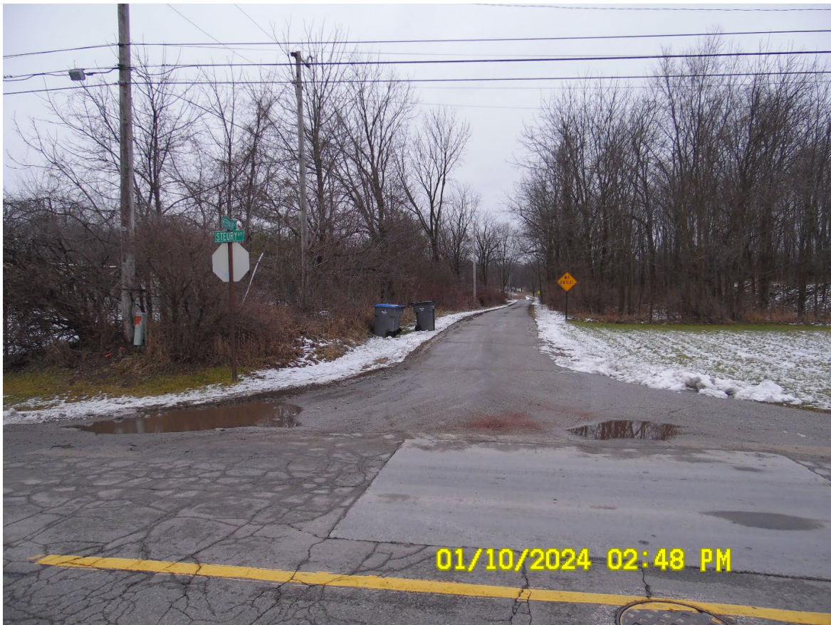
From Steury Avenue, looking east
