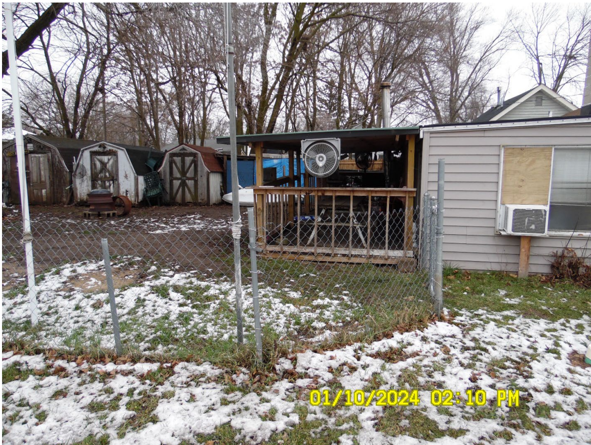
Looking north at the unapproved porch addition
