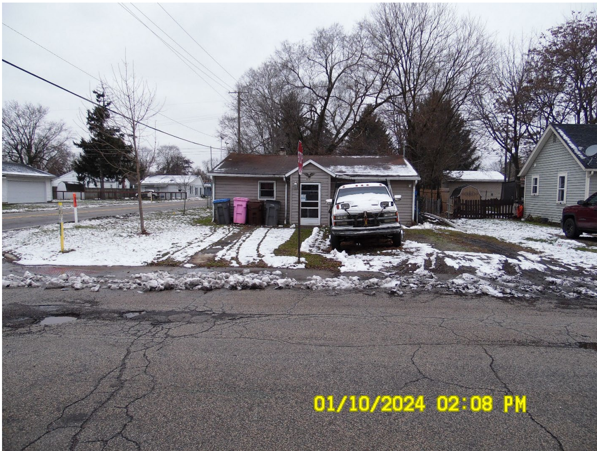
From 14 th Street looking west at front of home
